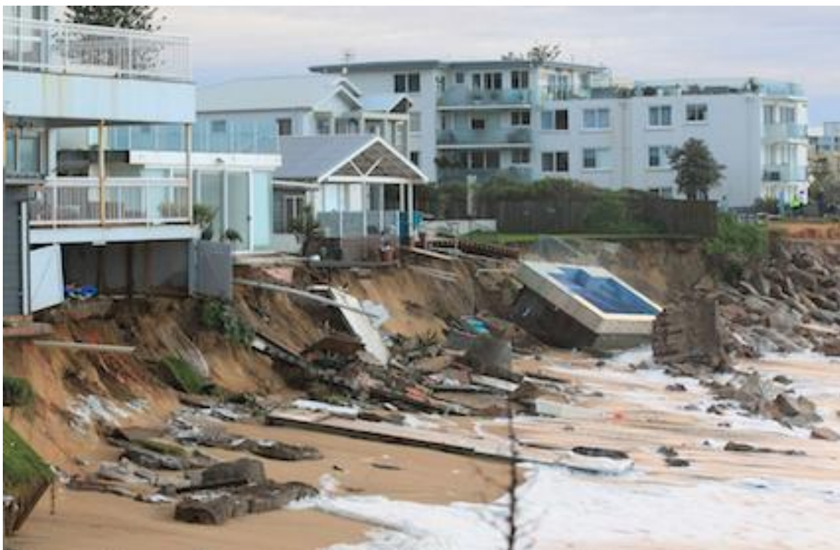
Figure 5.55 Image of damage caused at Collaroy Beach, Sydney, NSW during the June 2016 East Coast Low used in the survey. (Image: Peter Rae, 2016).
