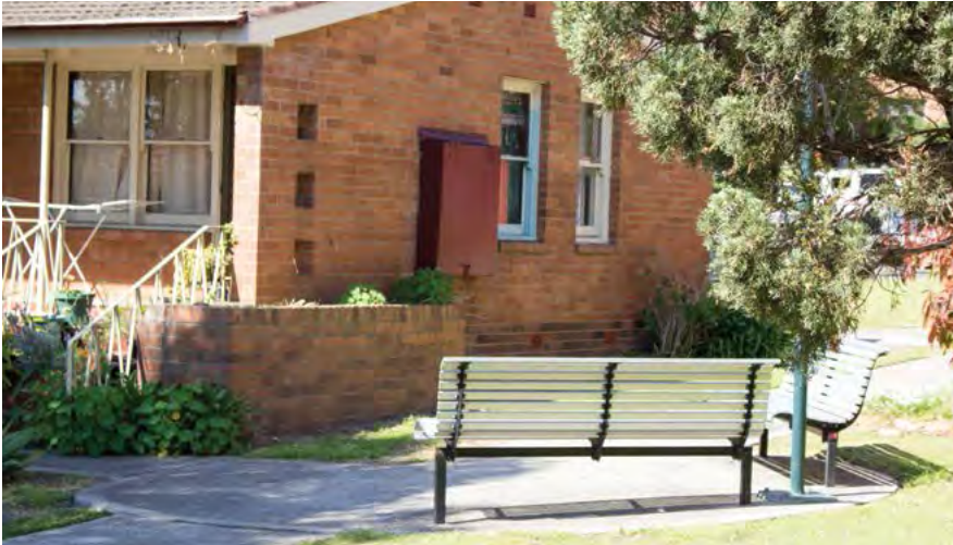
○ South Coogee Housing Estate
