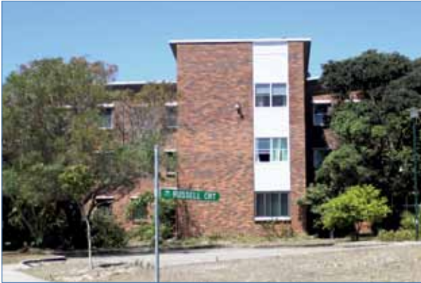
South Maroubra Housing Estate (photo: Kelli Ng)
