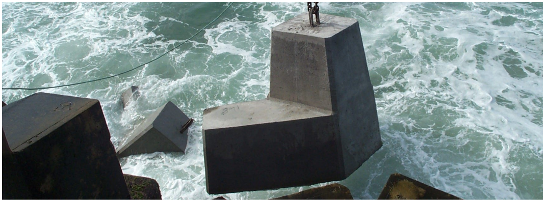
Figure 12: Placement of a Hanbar Armour Unit at Coffs Harbour, NSW
