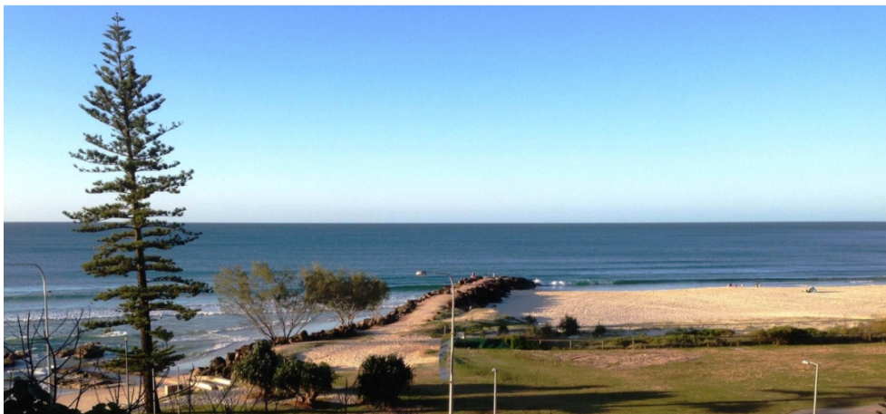
Figure 5: Kirra Point Groyne, Qld (Photo 07/07/2013, Prior to 2013 Restoration)
