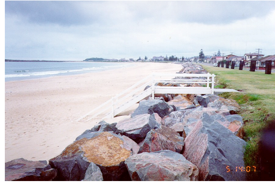
Figure 4: Rock Seawall Stockton Beach, NSW (Typical Pre-Storm Conditions)
