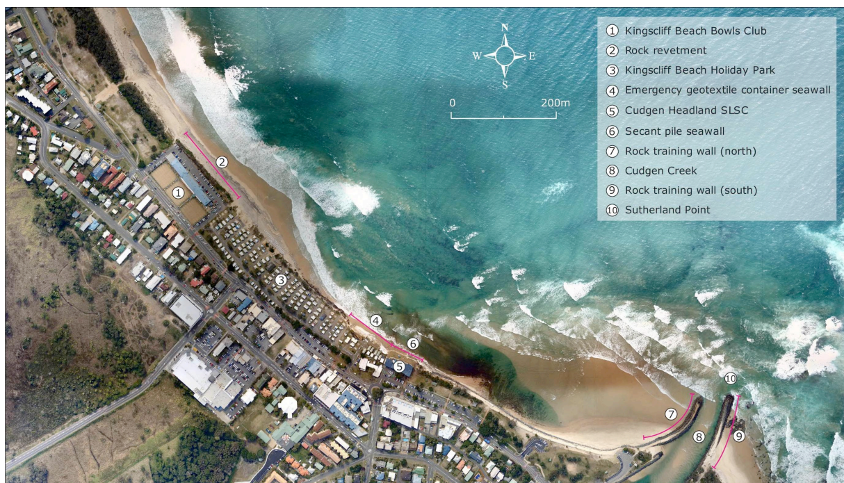
Figure 2: Site Details (Aerial Photo 21/07/2011)
