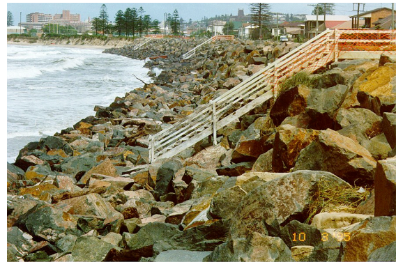
Figure 5: Rock Seawall Stockton Beach, NSW (Typical Post-Storm Conditions)
