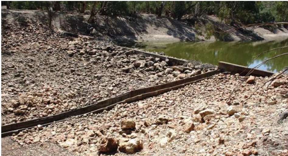
Figure 1.1 Upstream view of Weir 20A (WaterNSW, 2020)
