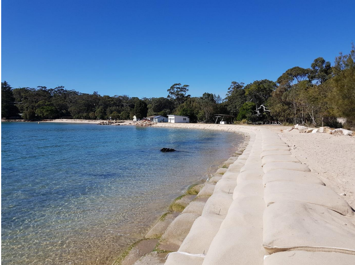
Figure 5.9 Example geotextile container revetment (0.75 m 3 containers at Bonnie Vale, NSW)
