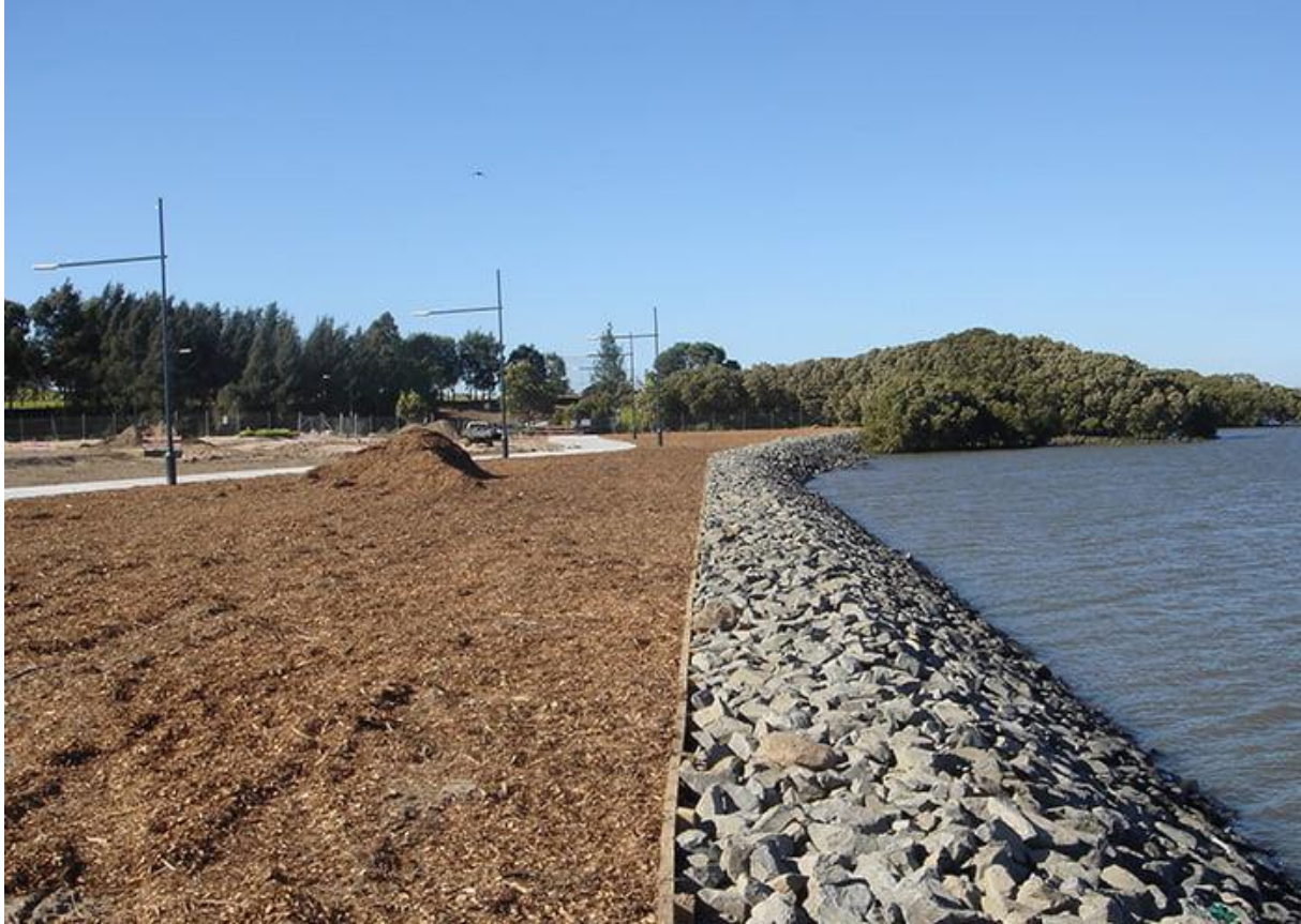
Figure 5.5 Example rock revetment (Ermington, NSW)
