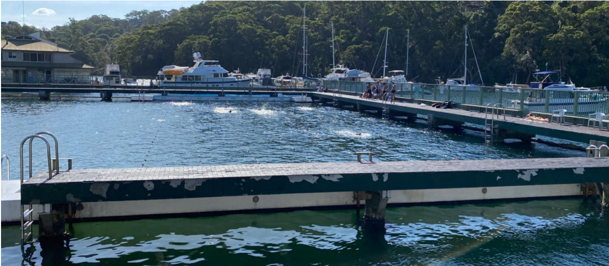
Figure 4.13 Pontoons and lane ropes – Northbridge Baths, NSW ( https://swimming.coffee/ )
