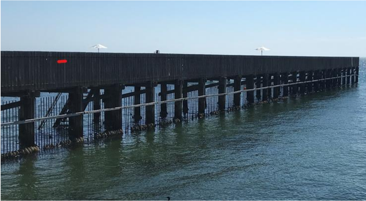
Figure 4.1 Timber and steel bar perimeter – Brighton Baths, VIC (James Carley)
