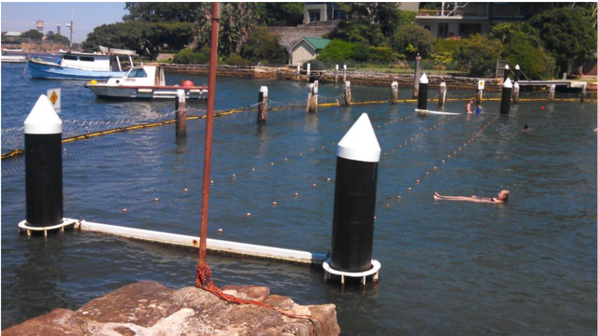
Figure 4.14 Floating turning boards for lap swimmers – Greenwich Baths, NSW
