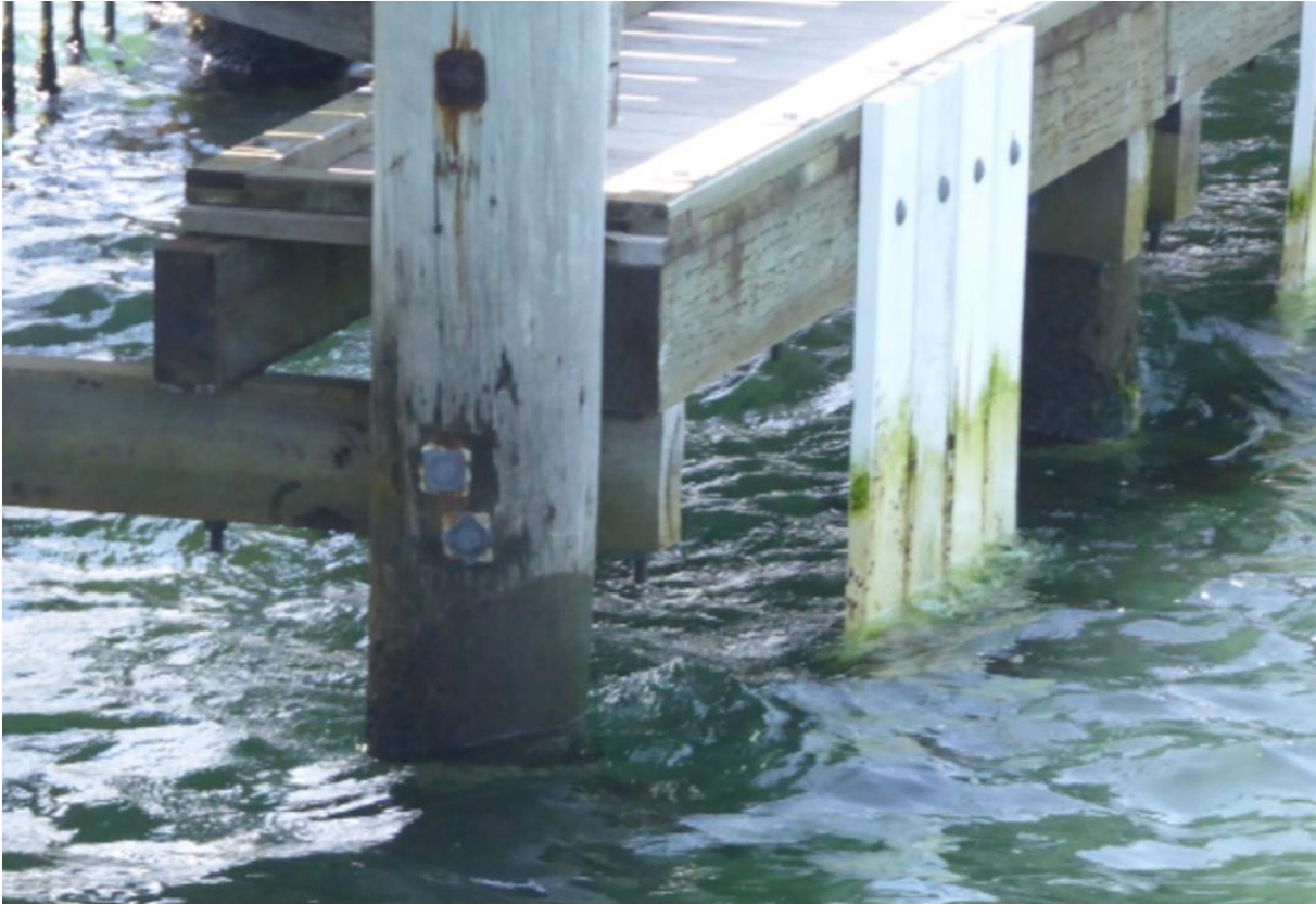
Figure 4.15 Fixed turning boards for lap swimmers – Brighton Baths, VIC
