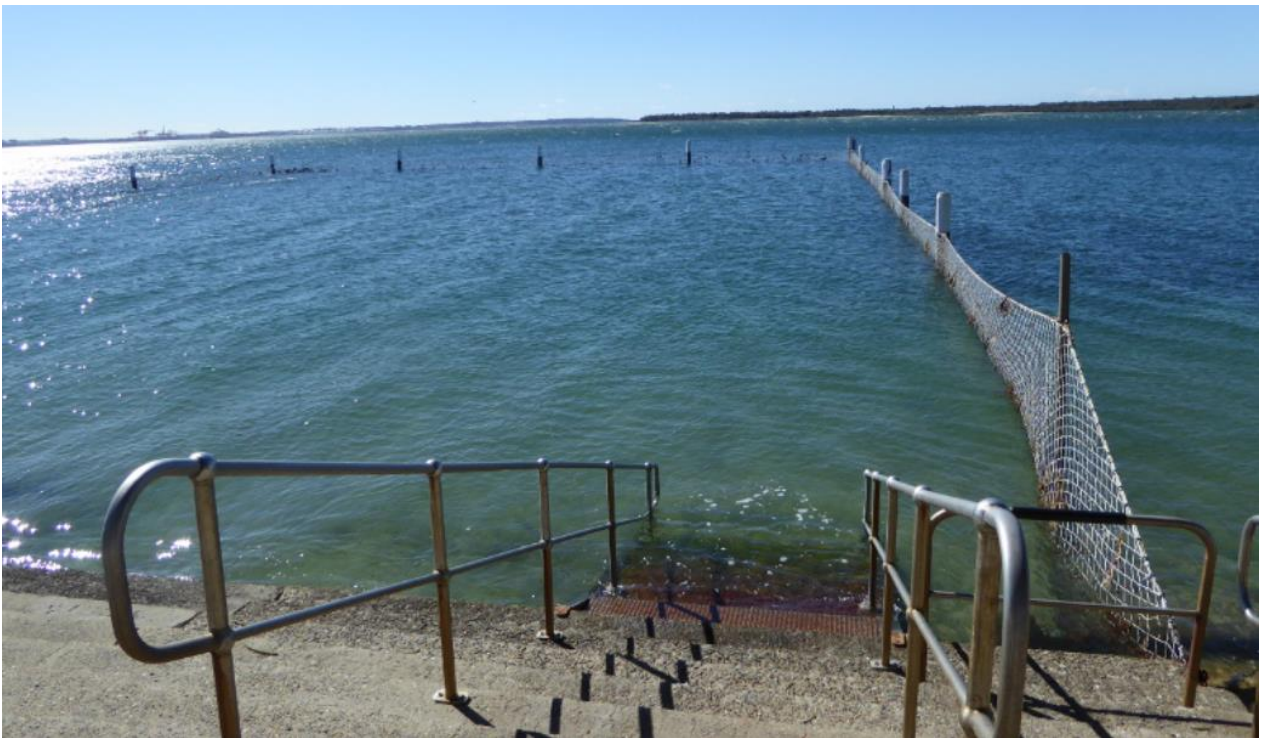
Figure 4.10 Net only enclosure – Vanston Baths, Sandringham, NSW ( oceanpoolsnsw.net.au )
