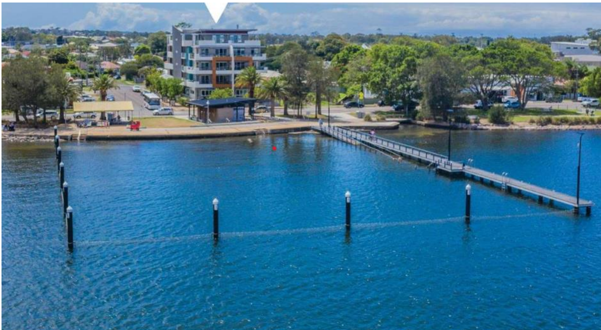
Figure 4.8 Single-sided walkway tidal pool – Belmont Baths, VIC ( homely.com.au )
