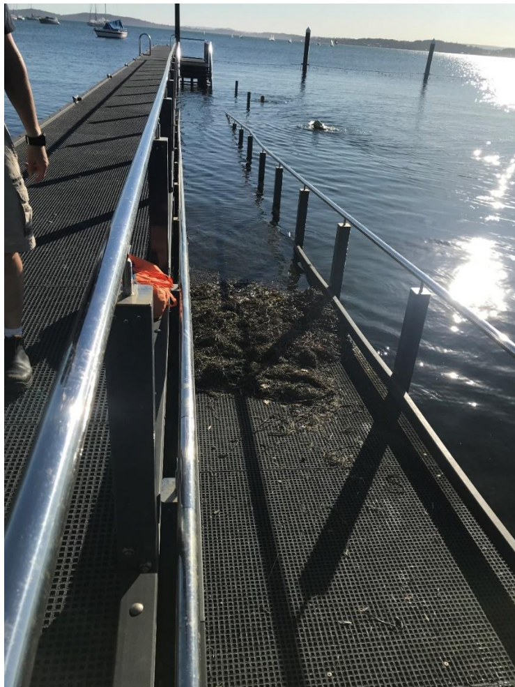
Figure 4.4 GRP walkway and ramp for people with low mobility into water – Belmont Baths, NSW (James Carley)
