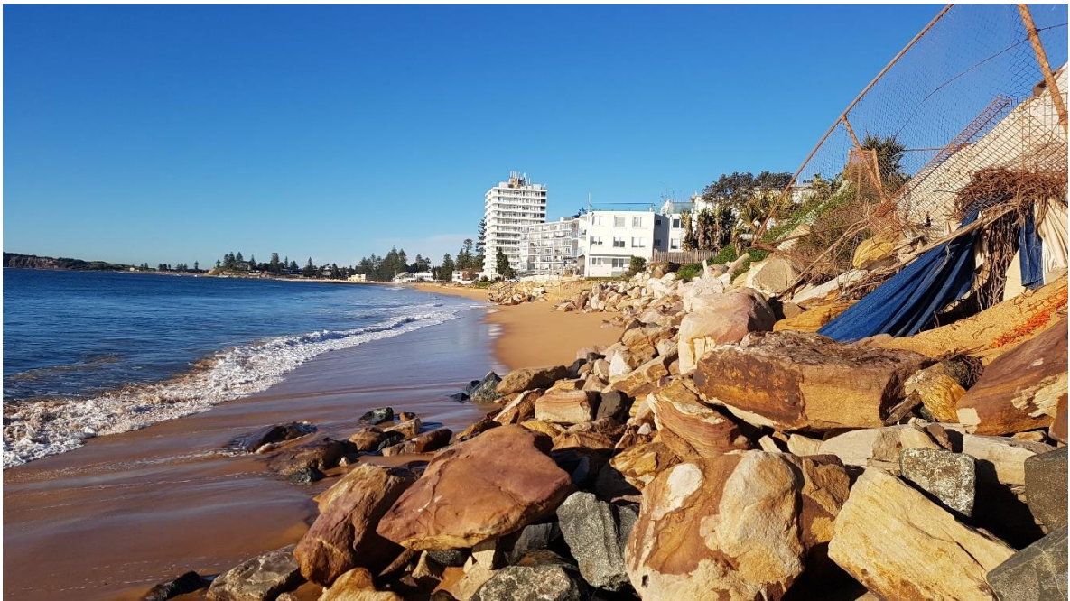
Figure 10: Erosion as seen from Wetherill Street looking south on 13 July 2018
