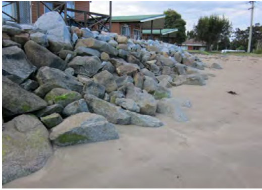
a) Eastern end of rock revetment wall
