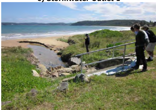
e) Stormwater Outlet 2
