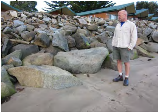
c) Rock wall armour properties are mixed
