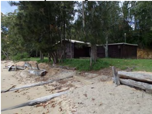
e) Wooden retaining wall at southern end
