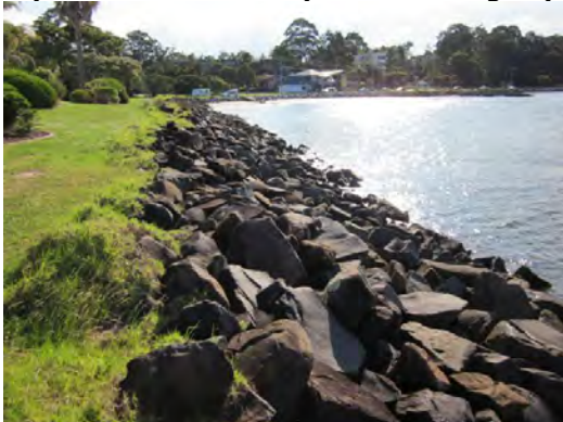
g) Eastern end of rock revetment wall
