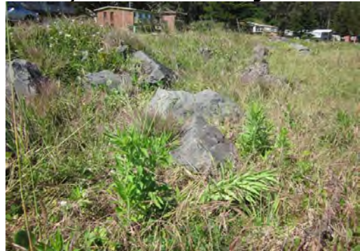
d) Partially buried rock revetment wall
