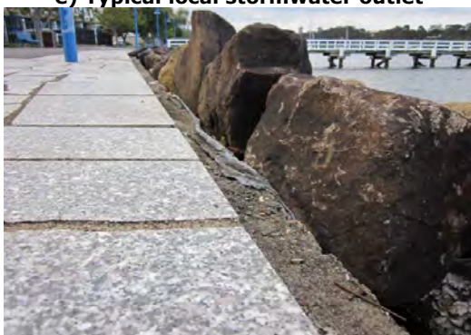
g) Geotextile underlayer visible
