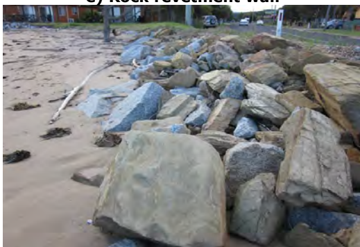
g) Rock wall armour properties are mixed
