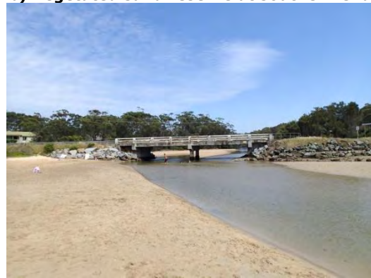
d) Beach Road bridge over Candlagan Creek
