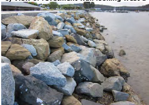
e) View of revetment wall looking west 2
