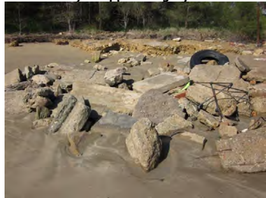
d) Building waste used as groyne armour
