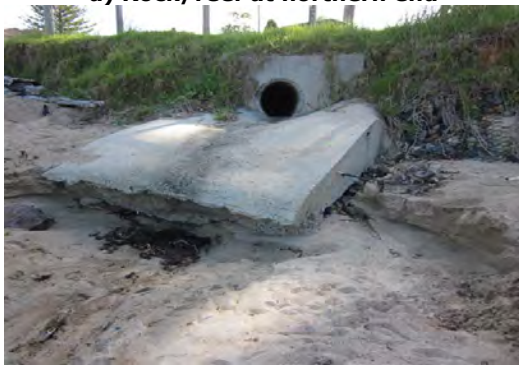
c) Stormwater outlet
