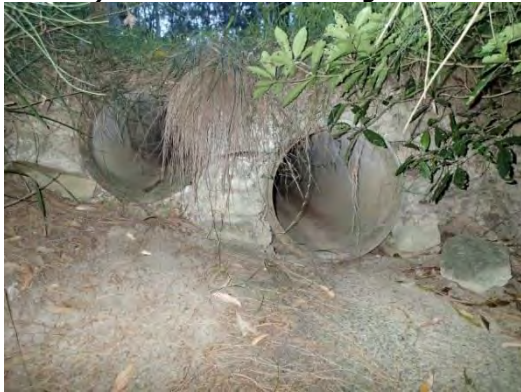
c) Stormwater outlets
