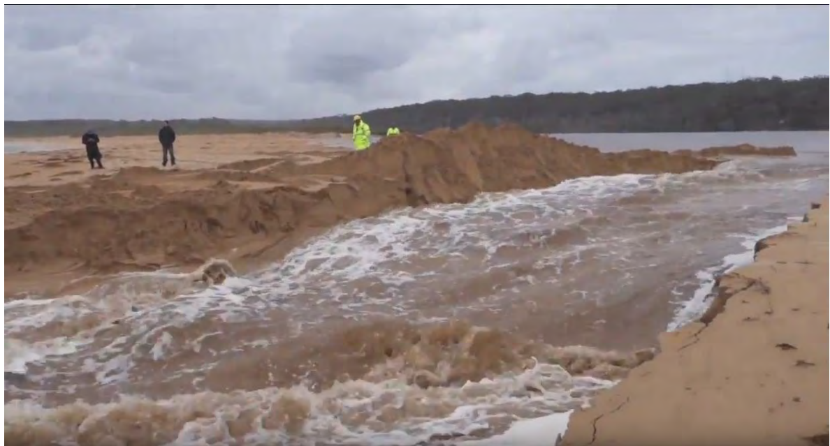
Figure M-1: Durras Lake Entrance Shortly After Mechanical Opening 26 August 2014 (Source: Durras Lake North Holiday Park, 2014)
