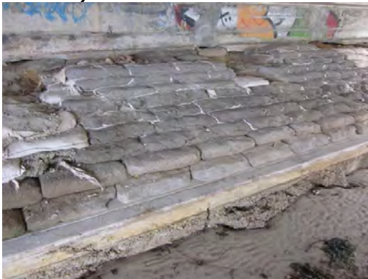
c) Scour protection at bridge abutments
