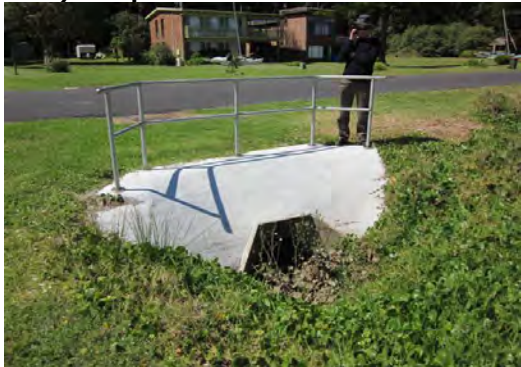
c) Stormwater Outlet 1
