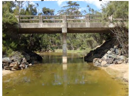
f) Durras Road bridge at southern end
