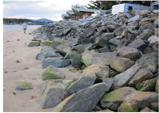
b) View of revetment wall looking west
