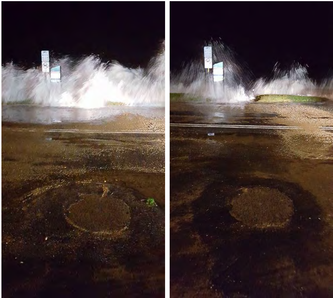
Figure 8-8: Overtopping at Intersection of Batehaven and Beach Road, 6/6/2016 10:00 pm (Source: Facebook)
