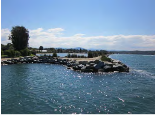
a) View of boat harbour looking west
