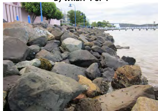
f) View of revetment wall looking north
