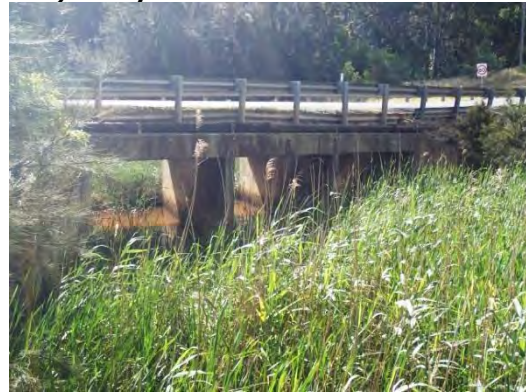
f) Box culverts under George Bass Drive
