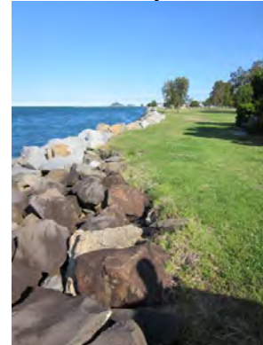
h) Western end of rock training wall
