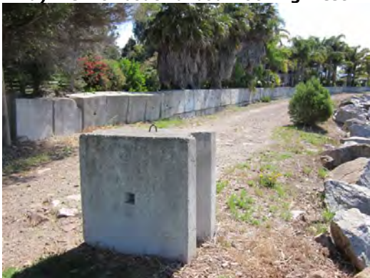
c) Concrete cube wall seaward of development
