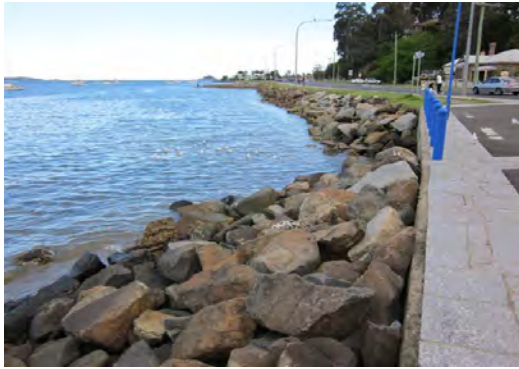
a) Western end of rock revetment wall
