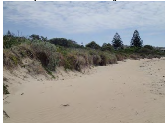
d) Scarp in the middle of the cove
