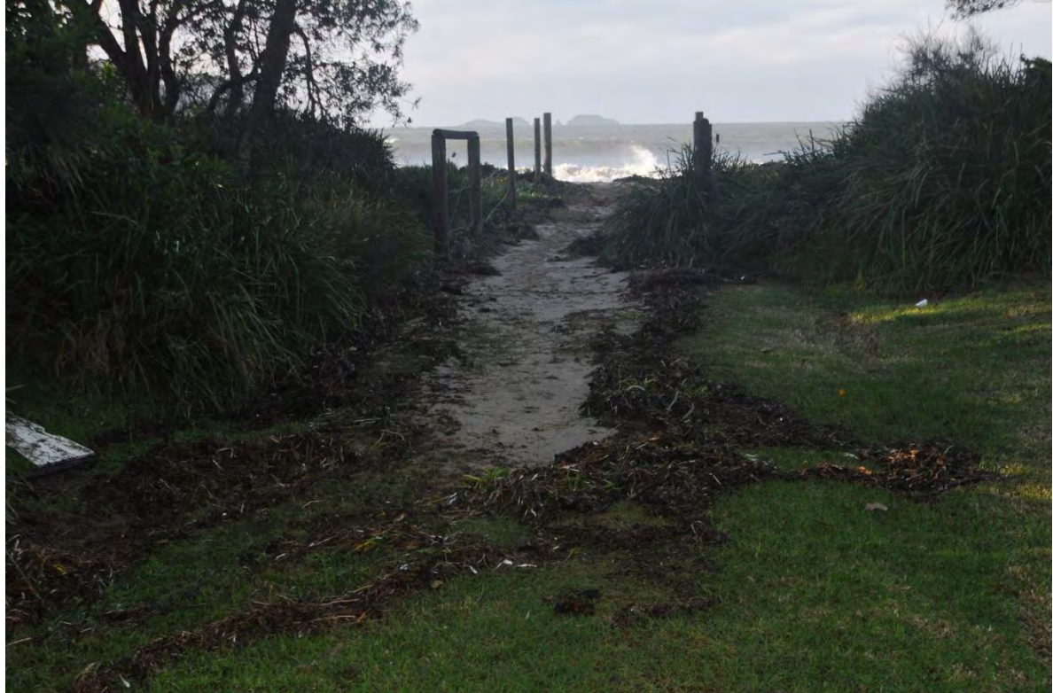
Figure 8-19: Inundation Debris Line at Surfside Beach (East), 6 June 2012 (Mr Lindsay Usher)
