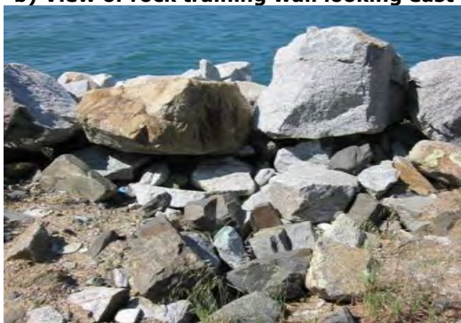
g) Typical secondary rock armour
