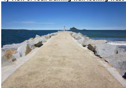
h) Eastern end of rock training wall
