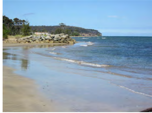
b) Unapproved groyne
