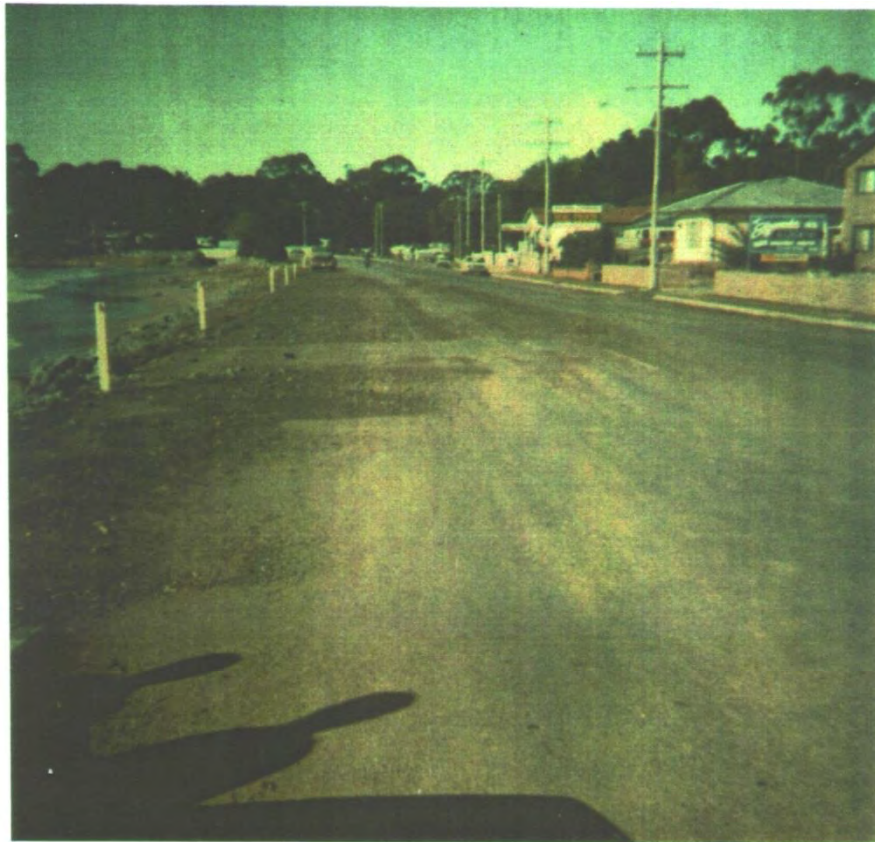
Figure 8-15: Overtopping of Caseys Beach Seawall 1 July 1984 (NSW PWD, 1989)
