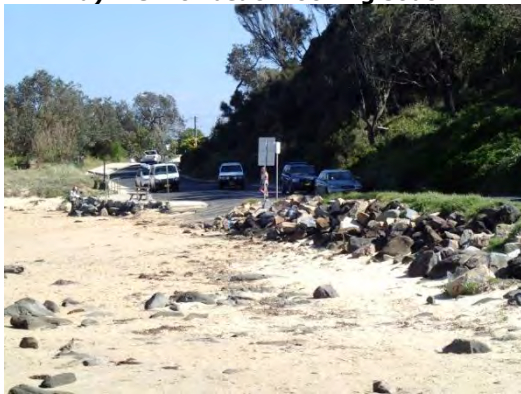
c) Boat ramp and rock revetment
