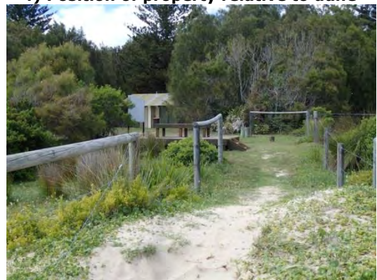
h) Formal access way and toilet amenities
