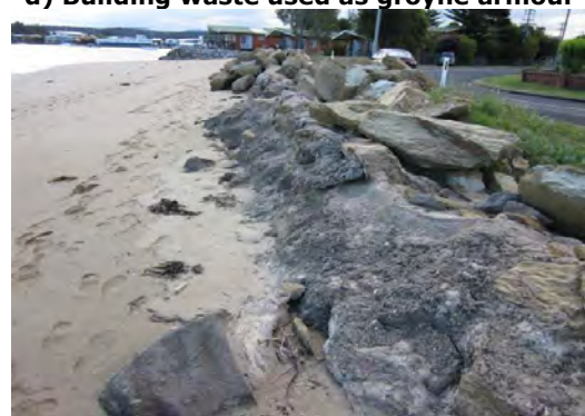
f) Wall armour is grouted together
