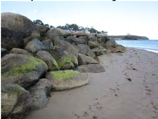
c) Rock armour at the head of the groyne
