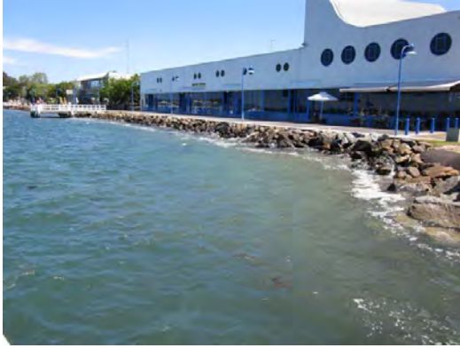
a) View of revetment wall looking south
