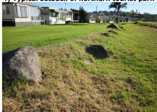
h) Predominantly buried rock revetment wall
