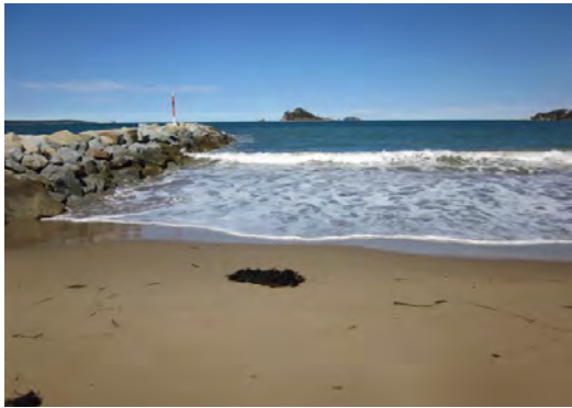
a) Training wall at northern end of beach
