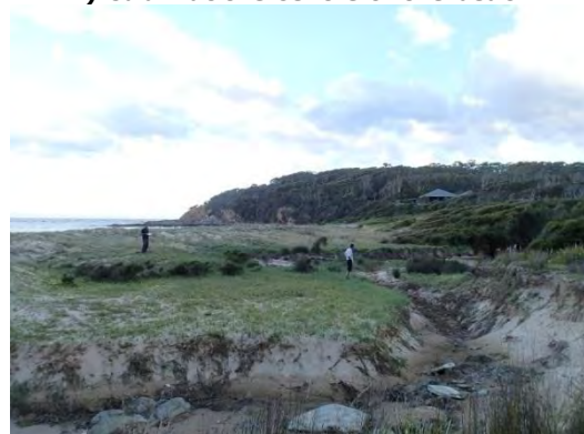
g) Scour of the banks of the creek
