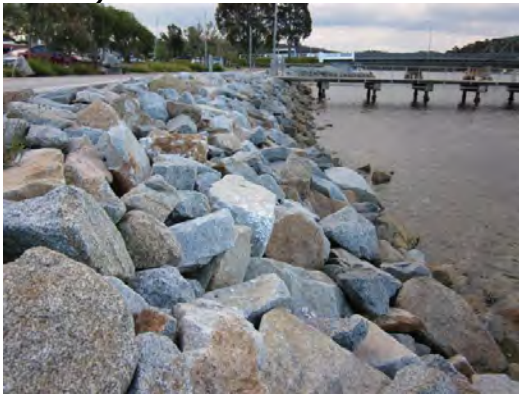
c) View of revetment wall looking west 1
