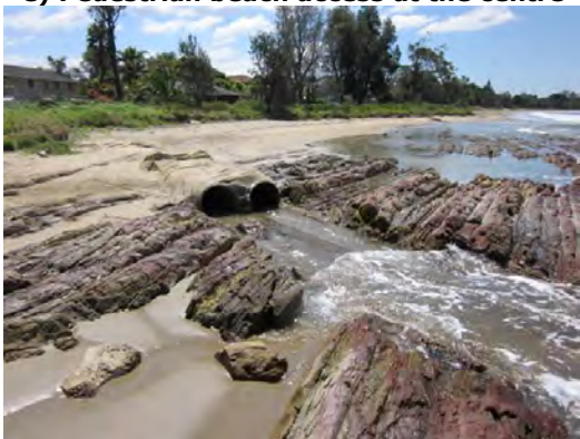
g) Stormwater outlet at southern end
