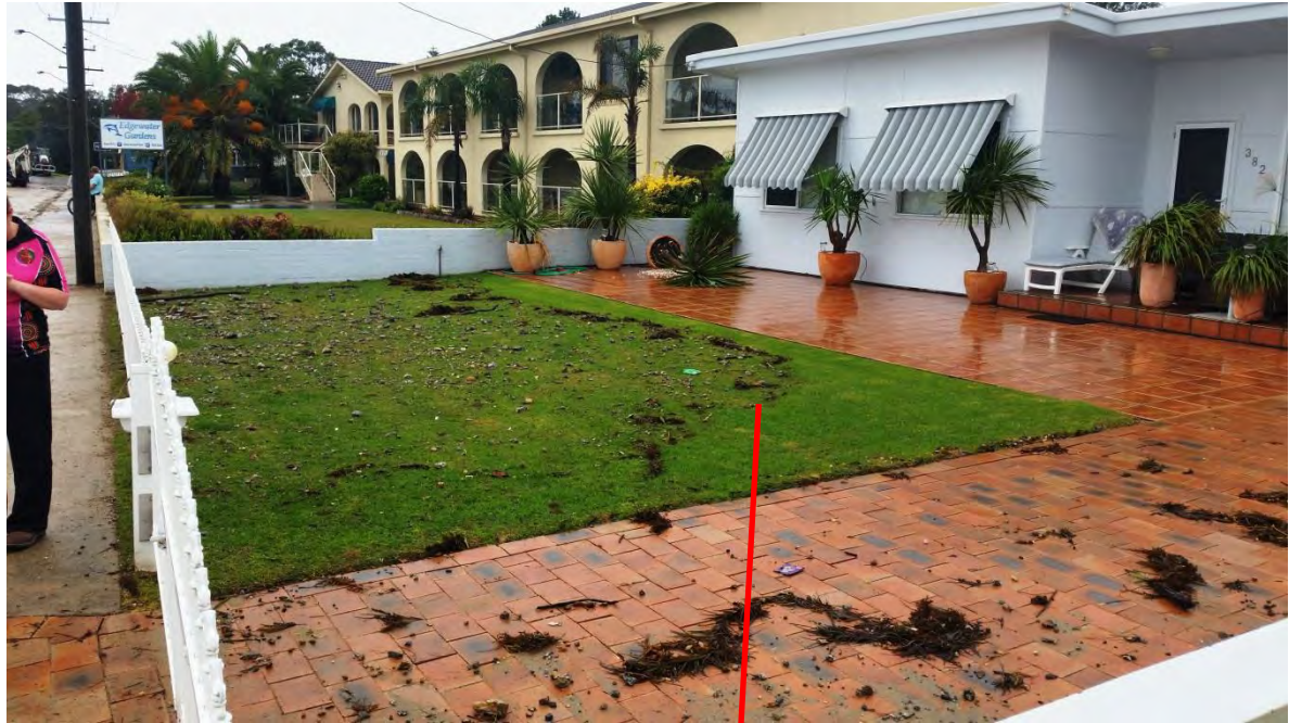
Figure 8-10: Runup Debris Line surveyed by WRL in the front yard of 382 Beach Road (ESC, 2016)
