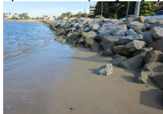
d) Revetment rock armour type 2 of 2
