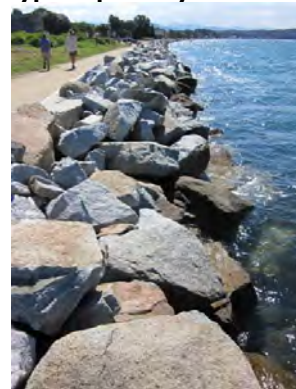
f) View of rock training wall looking west
