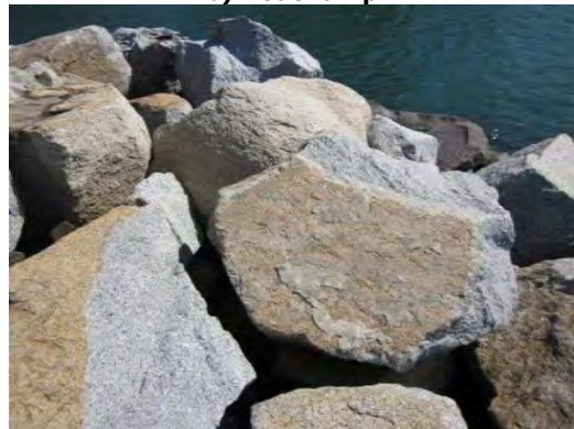
d) Typical primary rock armour
