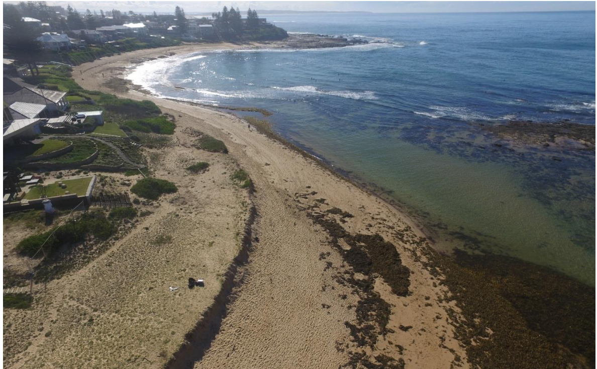
Figure 4-17: Blue Bay salient looking north. Note the significant weed build-up and dune scarp
