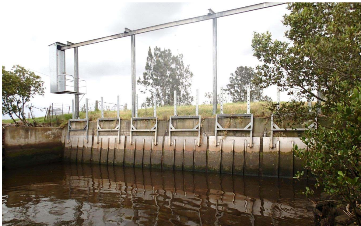
Figure D.2: P1 – Woodberry floodgates downstream
