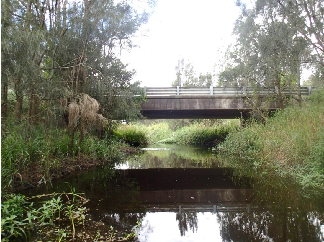
Figure D.5: P4 – Woodberry Road at Greenways Creek
