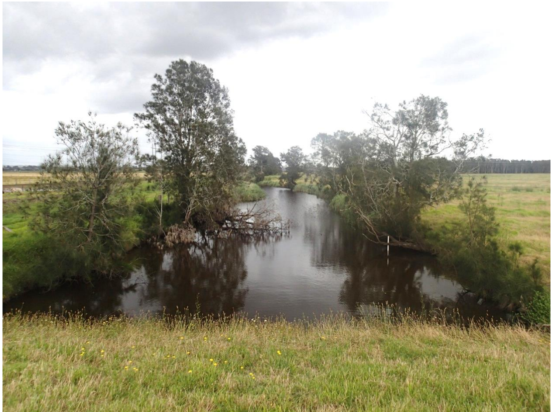
Figure D.4: P3 – Greenways Creek looking upstream from floodgates
