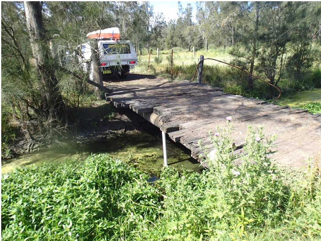
Figure D.12: P11 – Water level logger installation on wooden bridge at Greenways Creek
