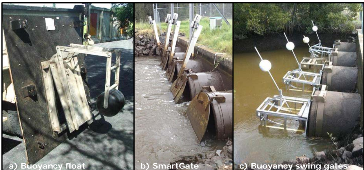
Figure 8.1: Different modified auto-tidal floodgate designs
