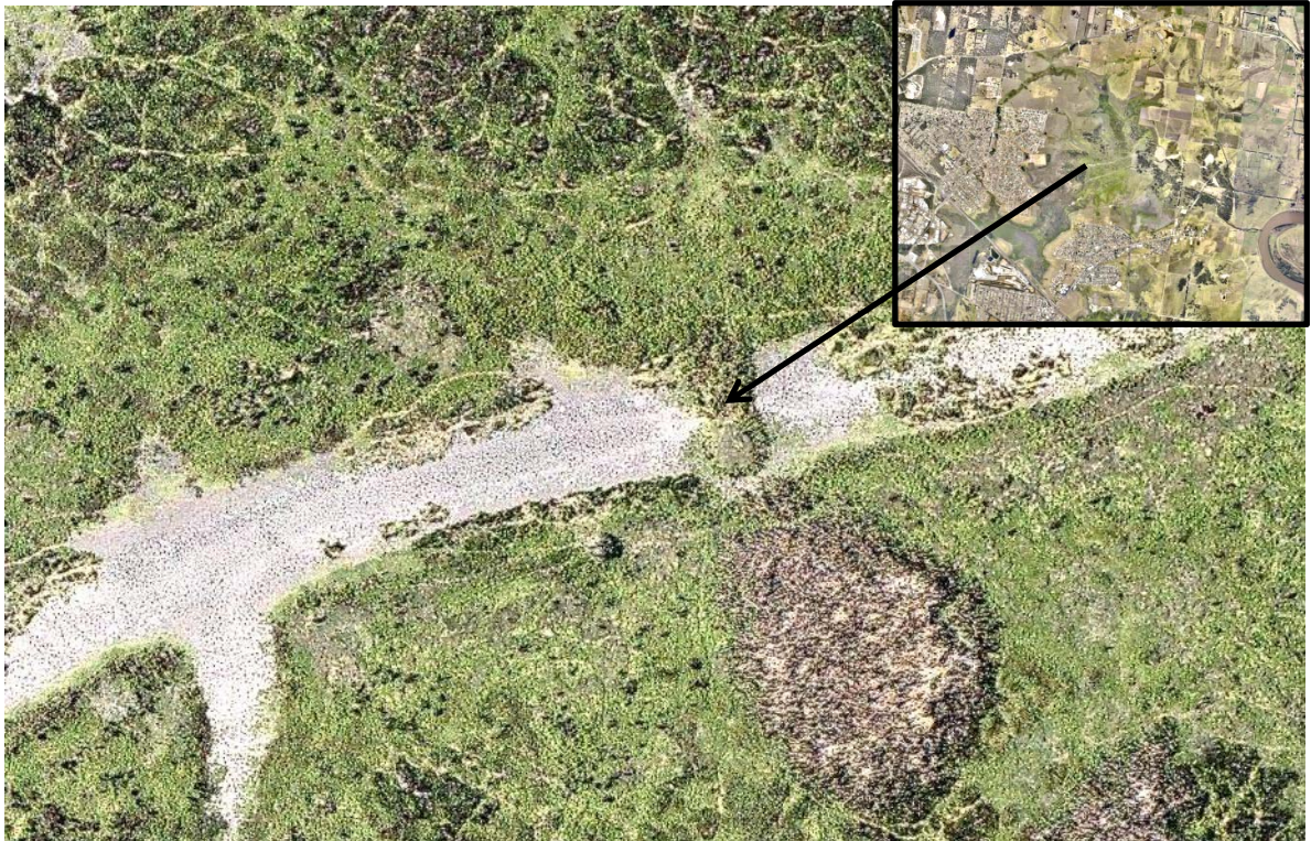
Figure 3.5: Collapsed culvert in the middle of the floodplain (Background image: Near Map)
