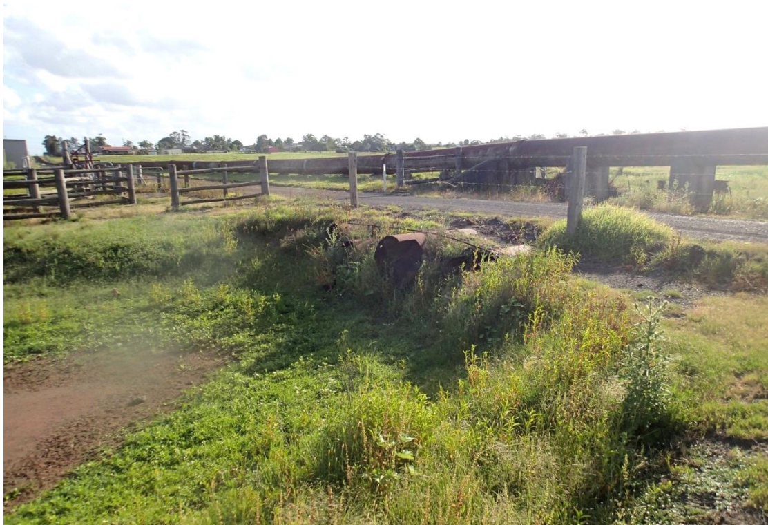
Figure D.8: P7 – Culverts under HWC pipeline access road
