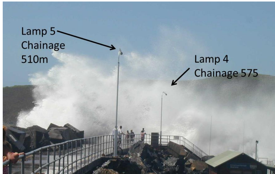
a) Overtopping Spray from Ch. 600 m to Ch. 700 m
