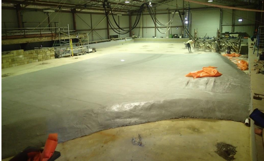
a) Overview of finished concrete bathymetry
