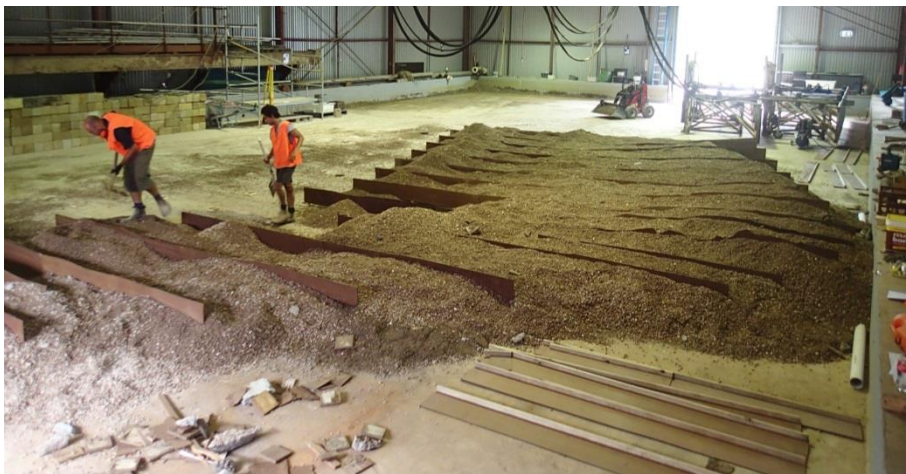
b) Aggregate being placed between Masonite Transects
