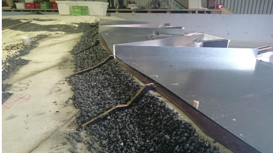
a) Overview of Existing Breakwater Core with Templates
