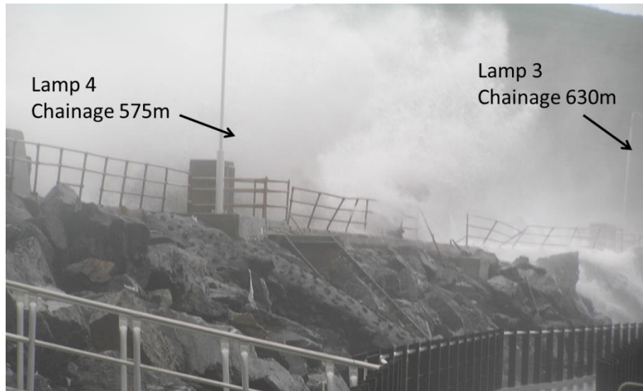
b) Example of Green-Water Overtopping around Ch. 600 m
