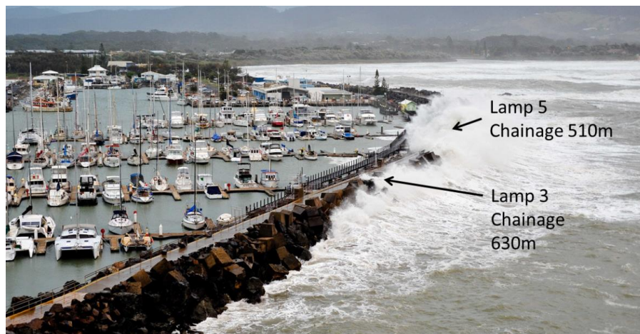
Figure 6.6: Observed Wave Overtopping from Muttonbird Island
