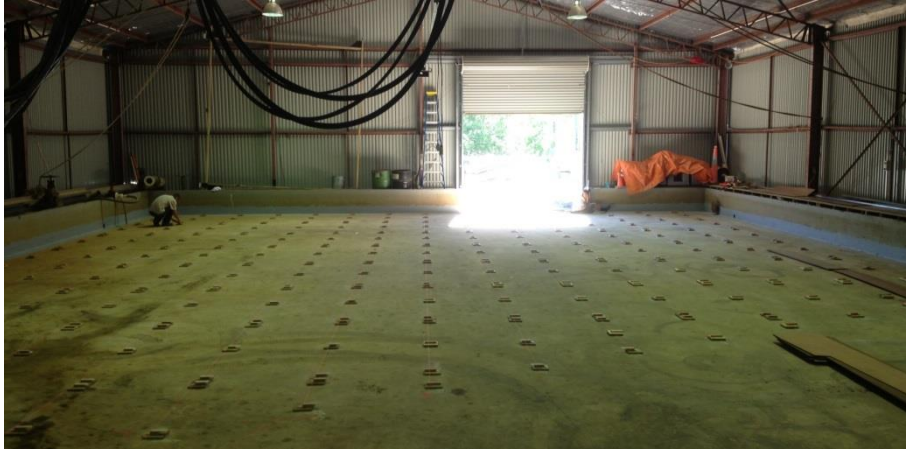
a) Preparation of Basin Floor
