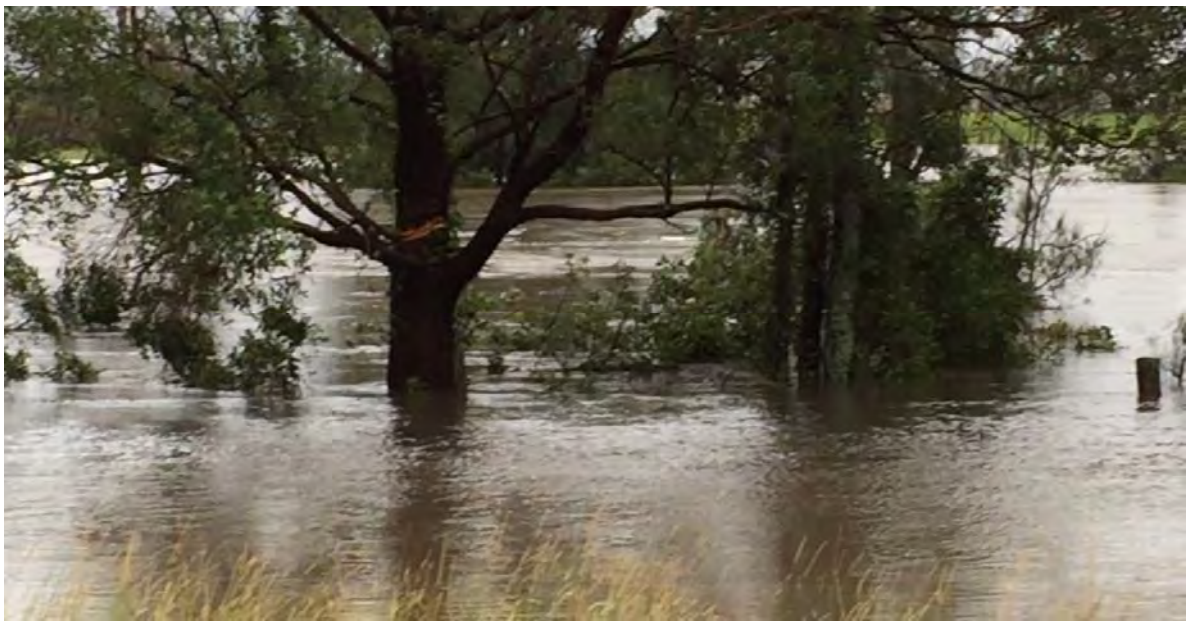
Figure 2-7: Images of April 2015 Flood on Seaham Weir Pool (Source: Mr John Spearpoint, 2015)
