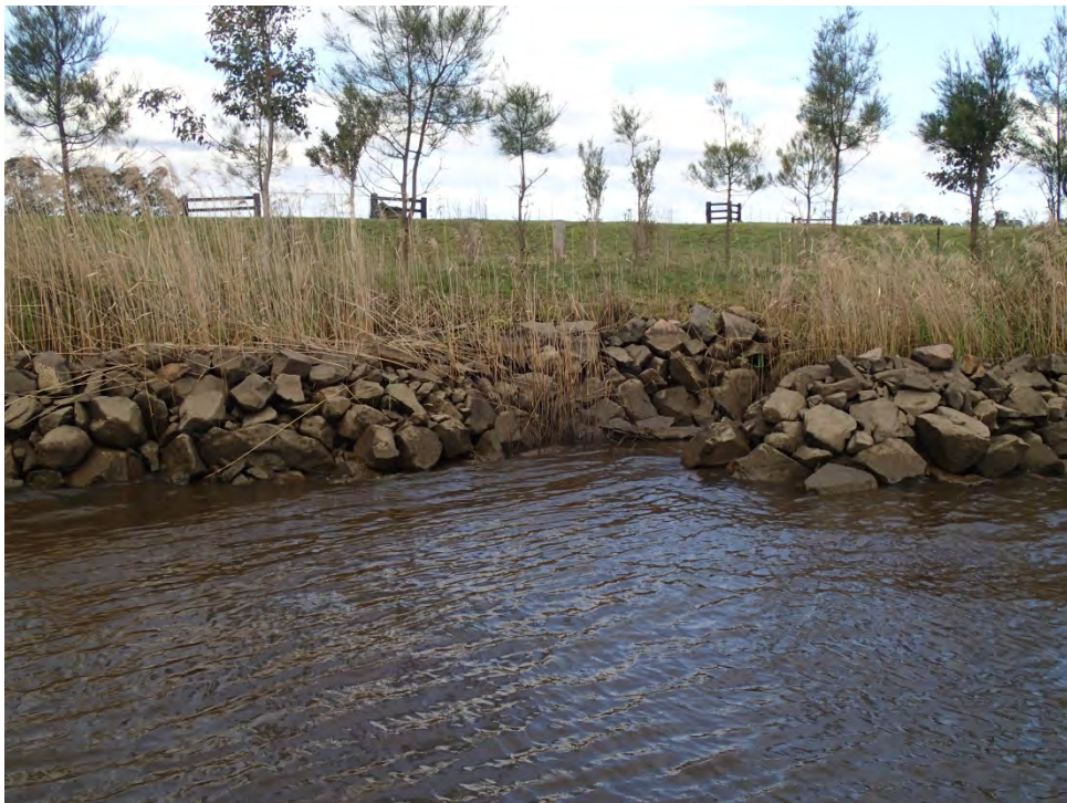
Figure 5-16: Rock Fillets at Transect R55C on the Lower Williams River (August 2015)
