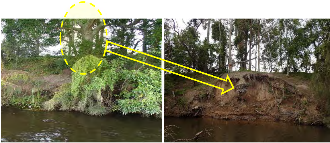
Figure 5-4: Comparison of March 2015 (Pre-Flood) and August 2015 (Post-Flood) at Site L11A
