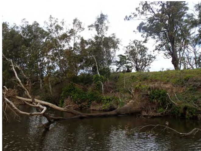
Figure 6-5: Riverbank Conditions Worsened at R04C From 'Mildly Resistant' in 2012 (Top) to 'Highly Erosive' in March 2015 (Middle), and 'Highly Erosive' in August 2015 (Bottom)
