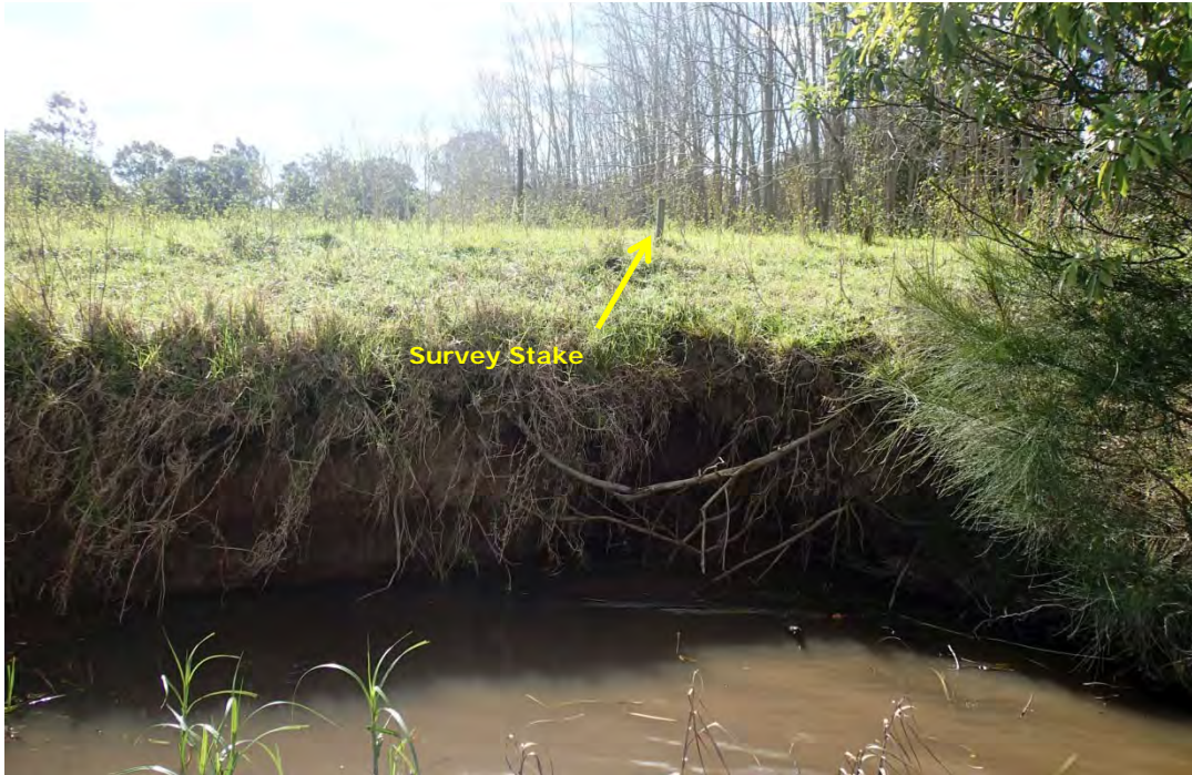
Figure R-4 : DLCS Monitoring Site 8 (August 2015)
