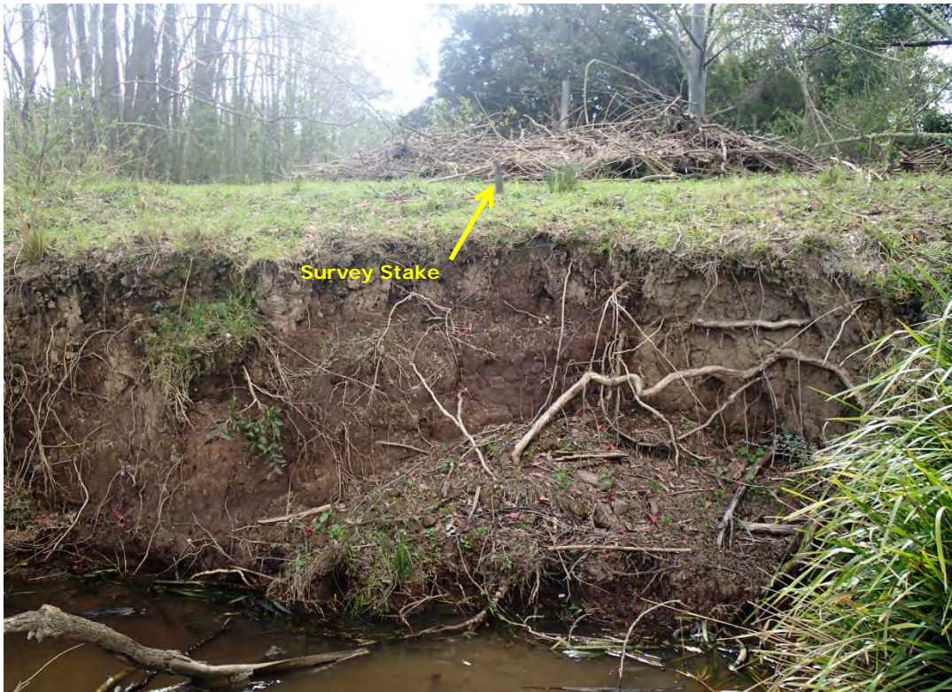
Figure R-5 : DLCS Monitoring Site 9 (August 2015)
