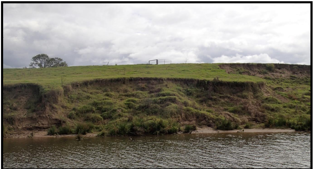
Figure 3-11: Significant Erosion, Slumping and Undercutting of Riverbanks where Stock Access is Present at Stretch L5
