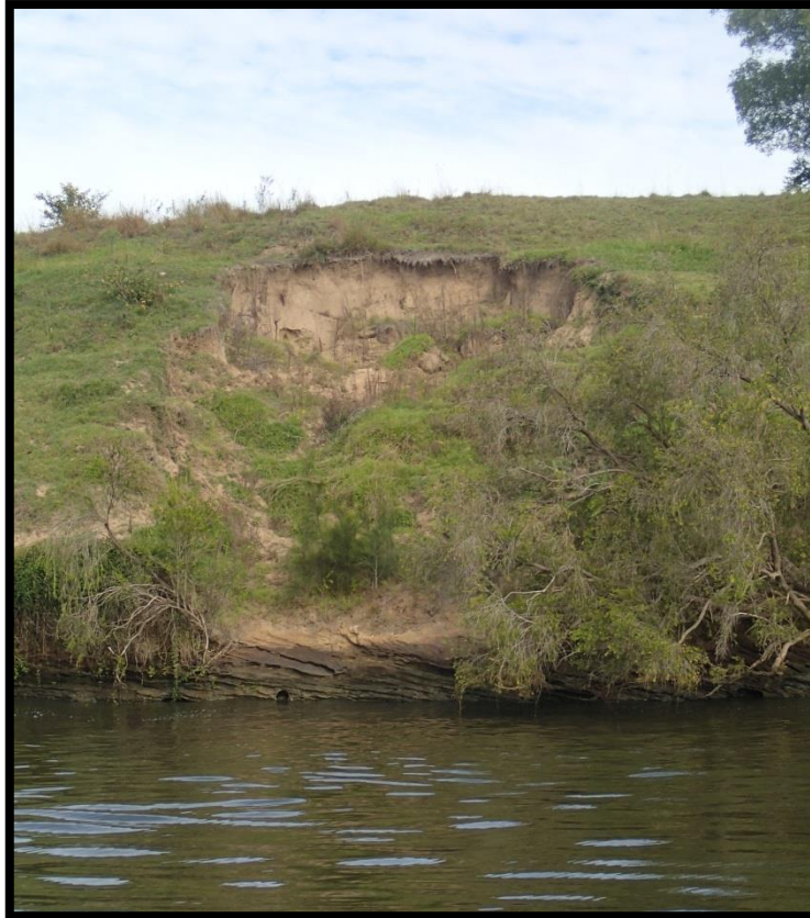
Figure 3-8: Erosion on Upper Bank Above Completely Armoured Wave Zone
