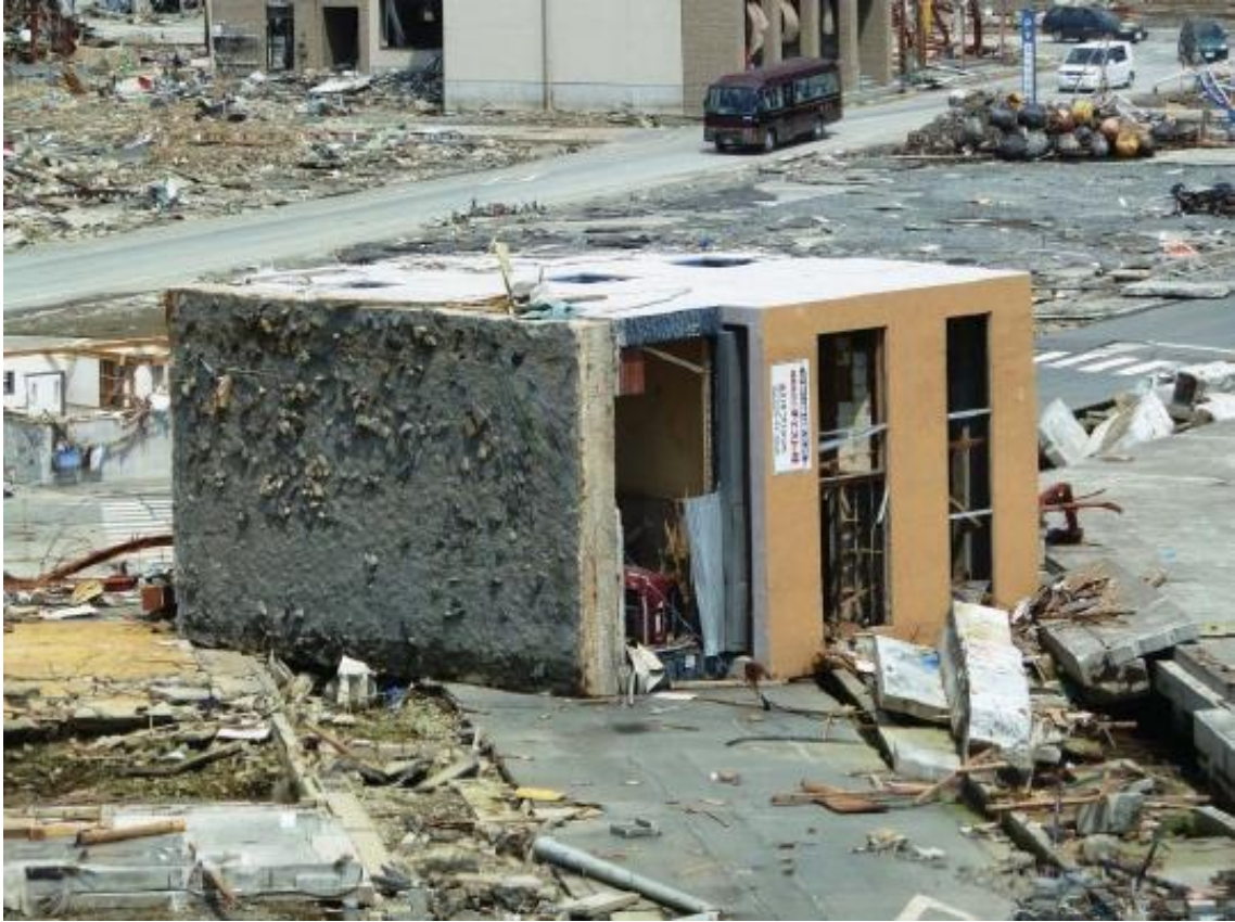
Figure 4-3: Overturned three-storey commercial building on mat foundation (Source: FEMA, 2012)
