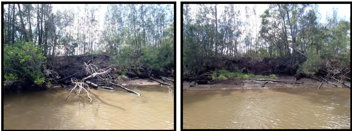
Figure 3-8: Significant Erosion, Slumping and Undercutting of Riverbanks where Stock Access is Present at Stretch L5
