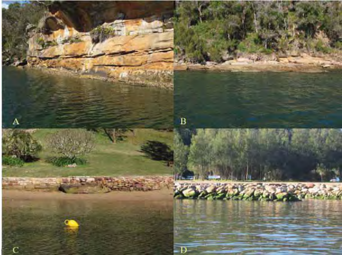
Figure A-2: Examples of Hard Surface Foreshore Classes in the Lower Hawkesbury Estuary. Natural Vertical Hard (A), Natural Horizontal Hard (B), Artificial Rock Walls (C and D) (Astles et al., 2010)
