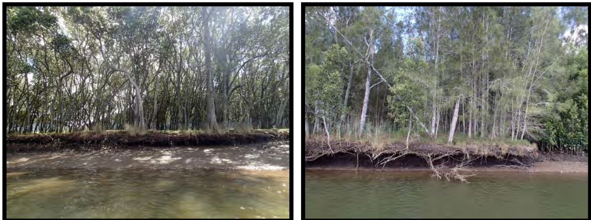
Figure 3-10: Significant Undercutting of Riverbanks where Stock Access is Present at Stretches L20 and R31
