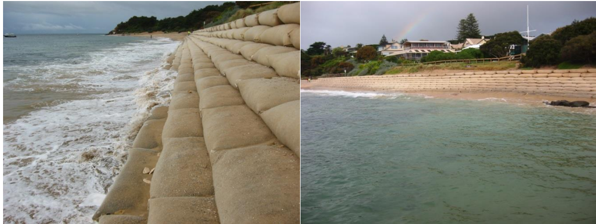
Figure 8.1: Typical Engineered Geotextile Container Revetment, Portsea, Victoria
