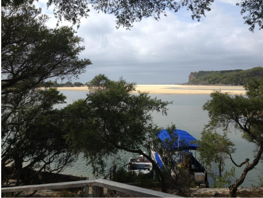
Figure 3.9: Vegetation and Landscaping at Top of Seawall
