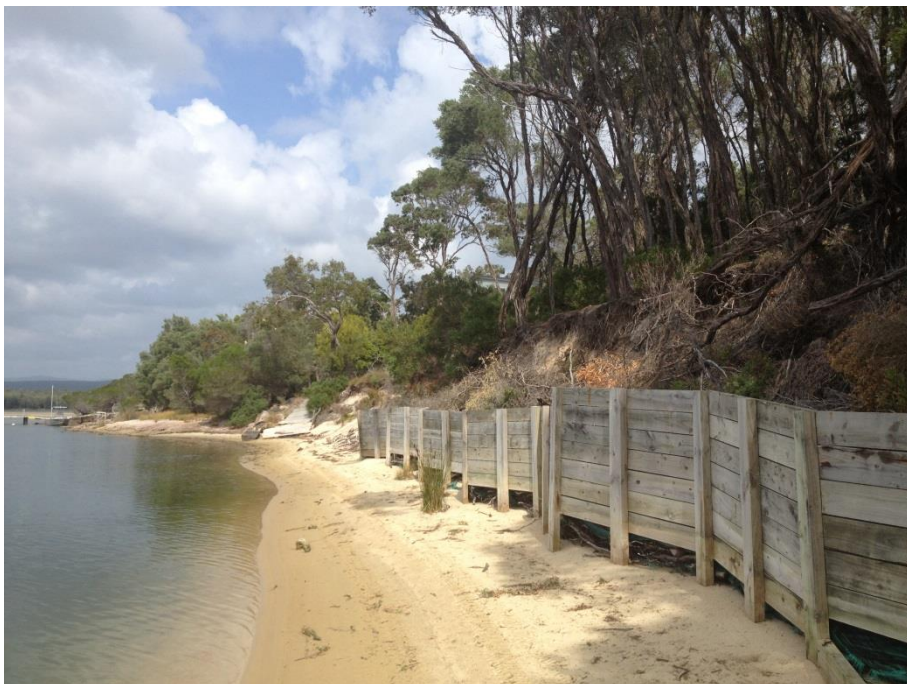
Figure 3.4: Existing Treated Pine Sleeper Seawall (Looking West)
