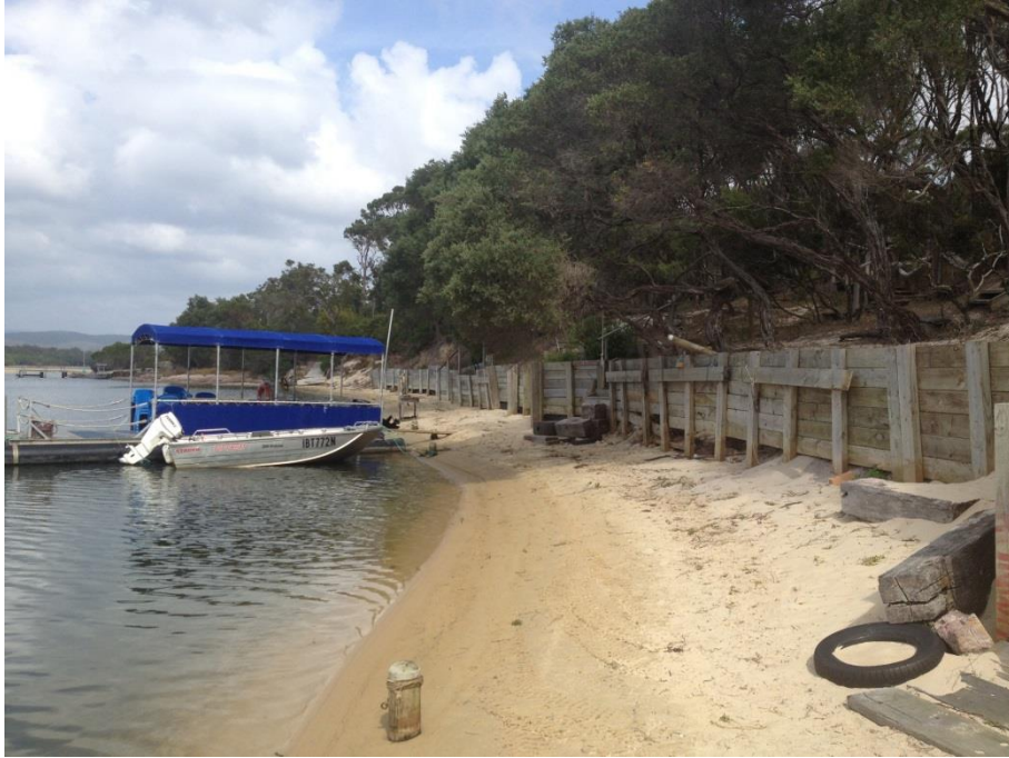
Figure 3.3: General View of Foreshore (Looking West)
