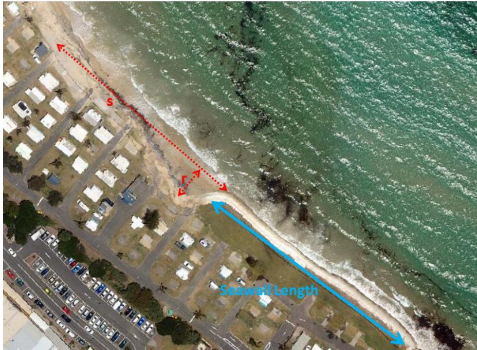
Figure 5.1: Kingscliff NSW Example of Excess Seawall End Erosion Depth, r and Length, s
