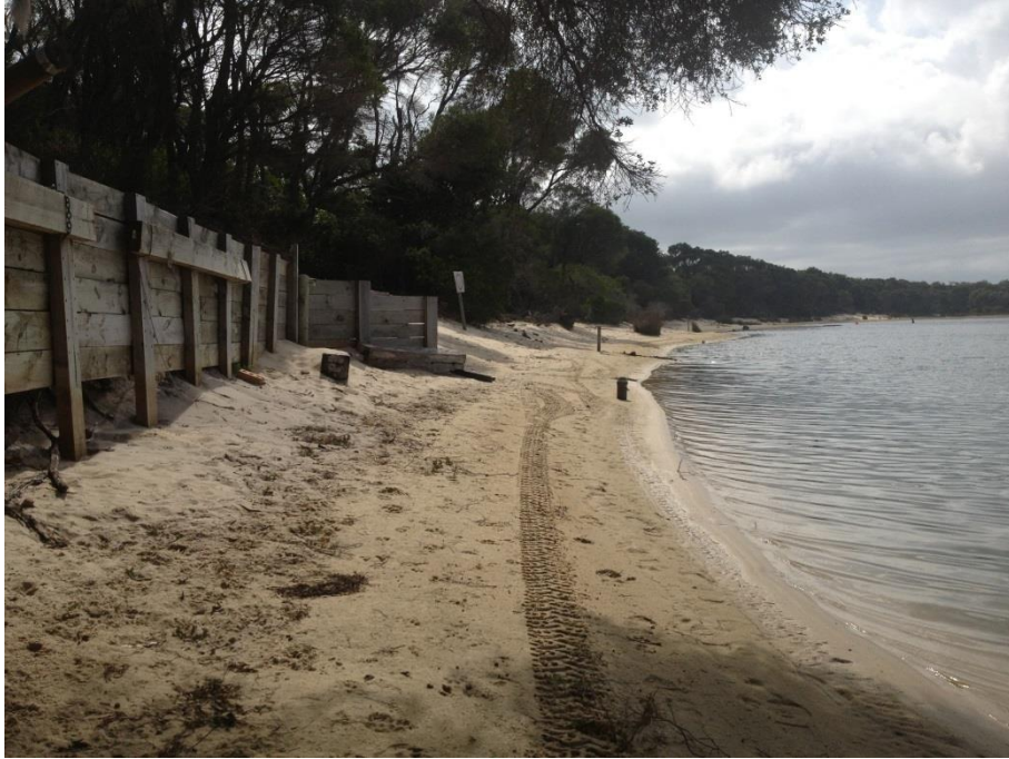
Figure 3.1 Site Foreshore Looking East
