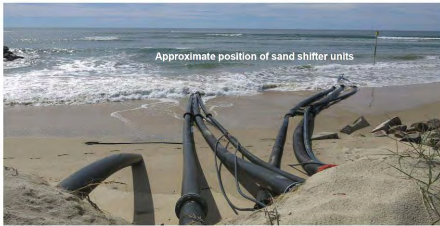
Figure 29.3: Sand Shifter during Operation (Source: SSM)
