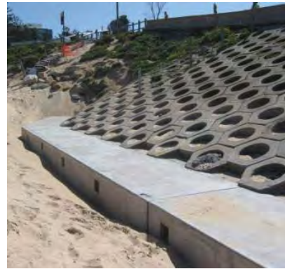
(b) Seabee concrete units (Sutherland Council)
