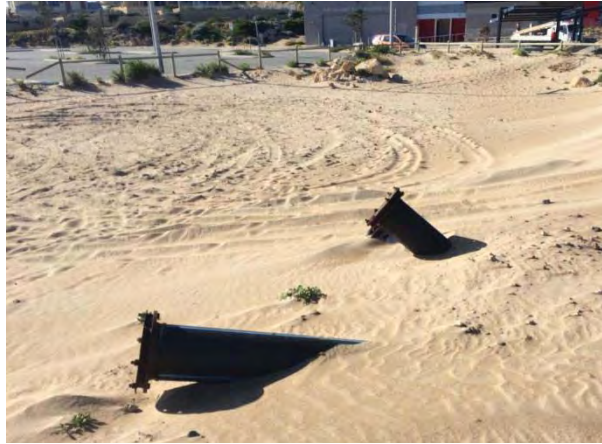
Figure 29.10: MSCU Associated Pipes when not in Operation
