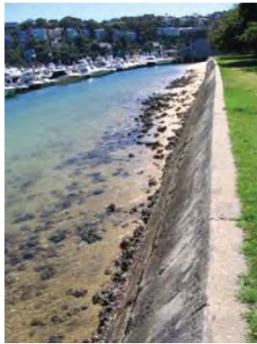
(a) Solid Concrete (Mosman Council)
