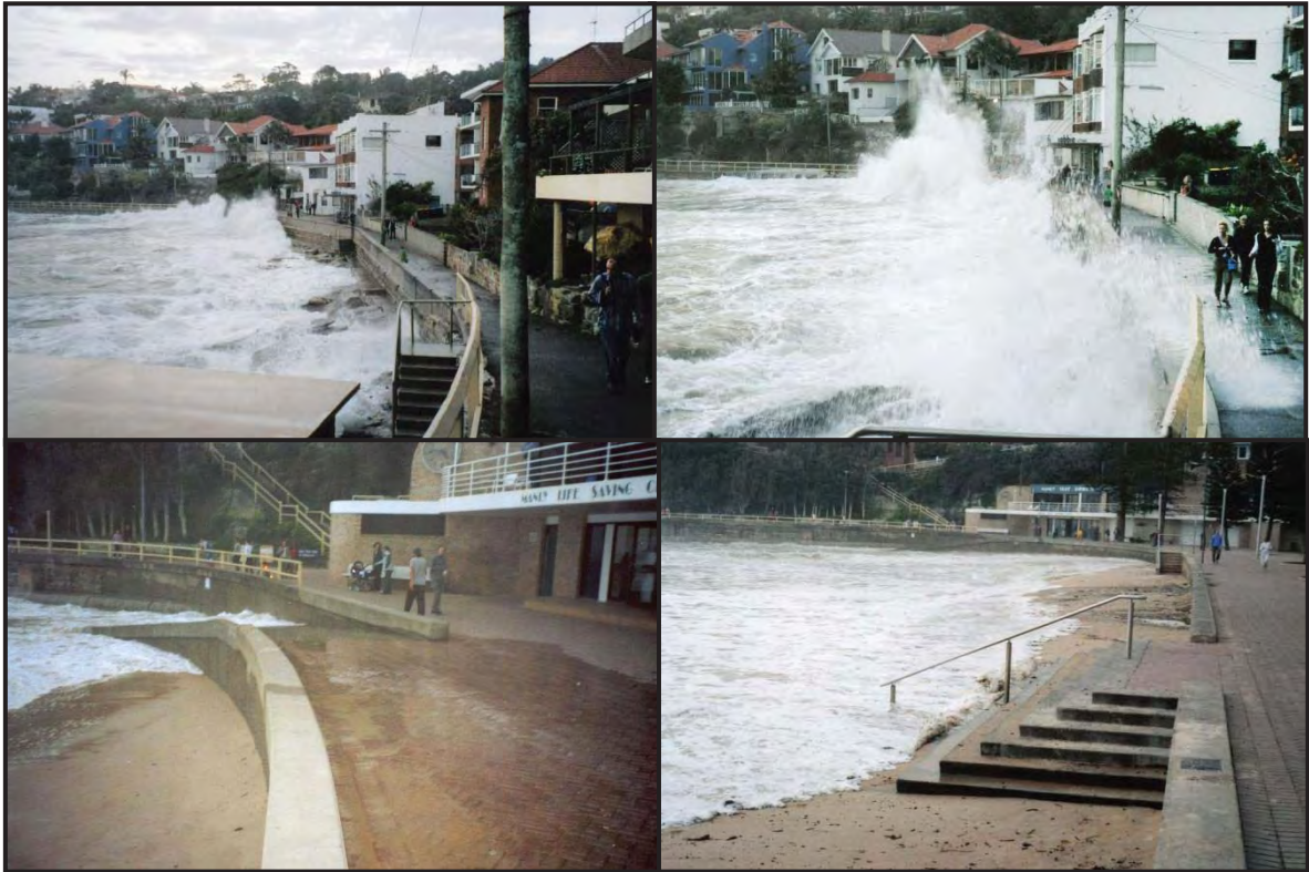
Figure 20.6: (Top) Wave overtopping the Manly to Shelly Beach seawall; (Bottom) Wave runup at Manly LSC boat ramp and Manly beach stairs (Victoria Pde). (Photos: James Carley WRL)
