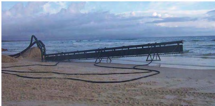
Figure 29.2: Sand Shifter Onsite before Installation/burial (Source: SSM)
