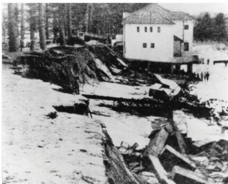
(a) Loss of promenade at Manly, 1950
