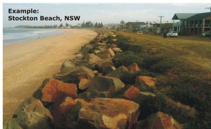
Figure 5.3: Terminal Seawall Alone
