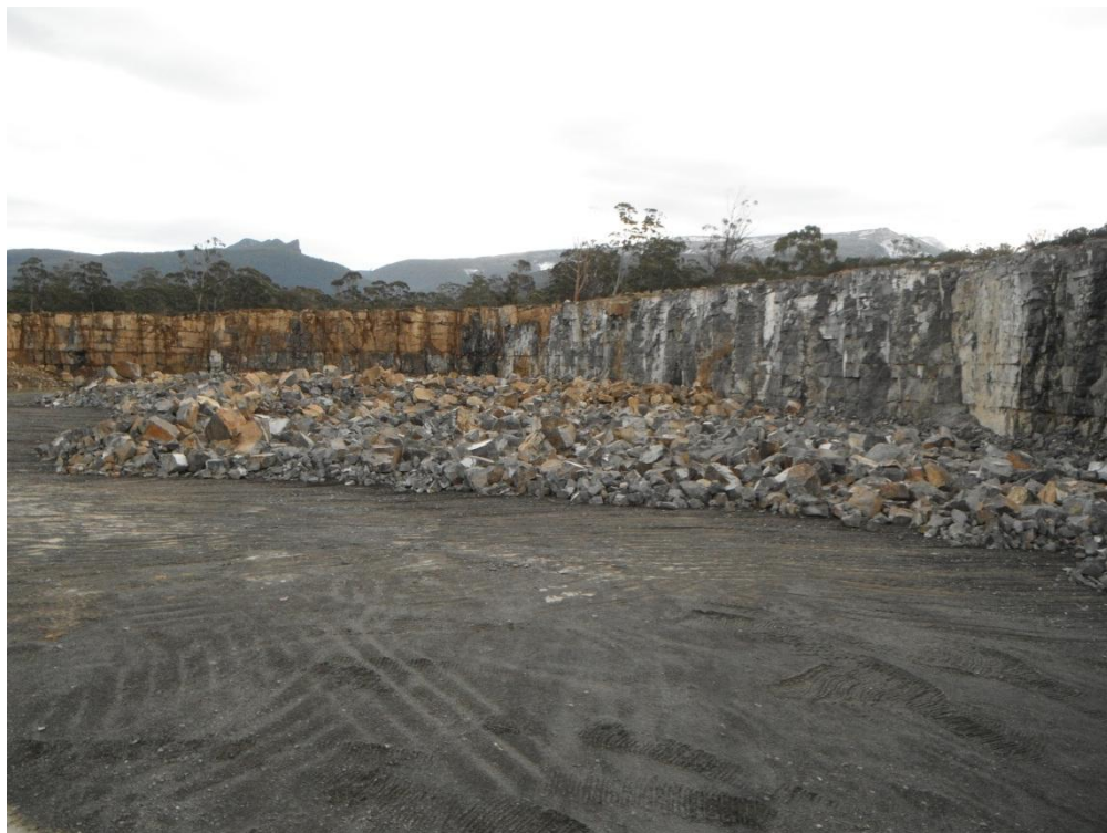
Figure 9: Dolerite Formation at Hazel Bros Quarry, Leslie Vale
