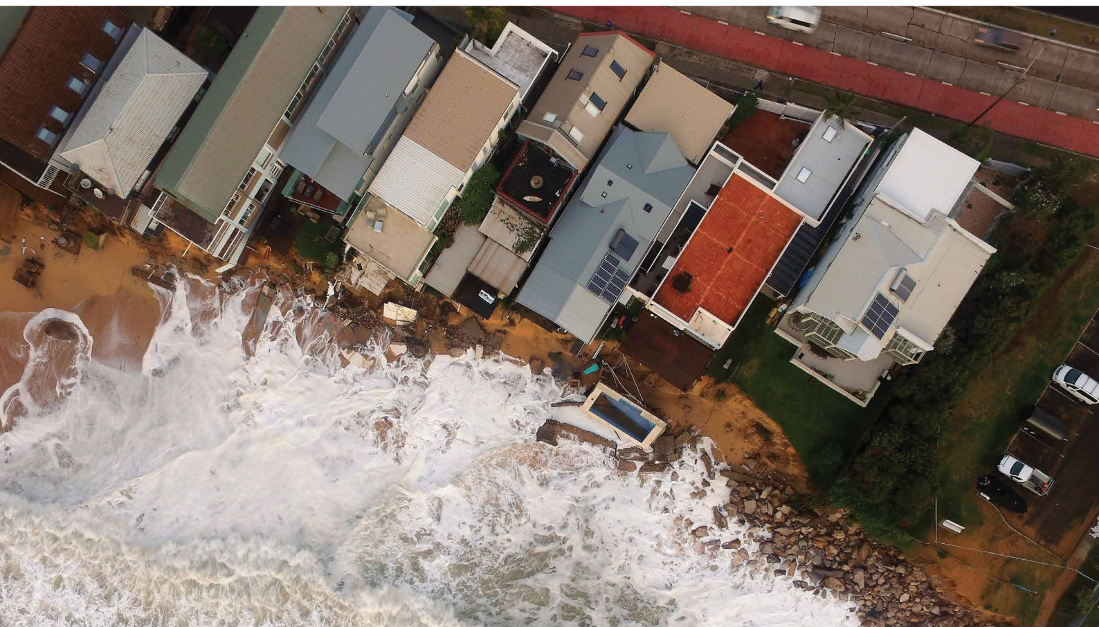
Coastal erosion during the June 2016 East Coast storm. Northern Beaches, NSW. Photo: Chris Drummond - WRL, UNSW
