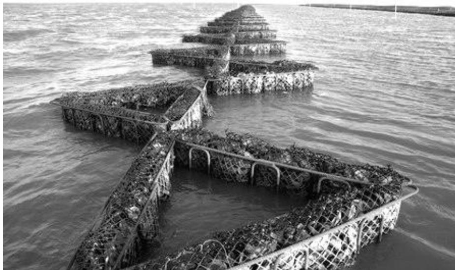
Figure 2.5 – ReefBLKs filled with oyster shells, installed at Coffee Island, Alabama, USA (Allen 2013)
