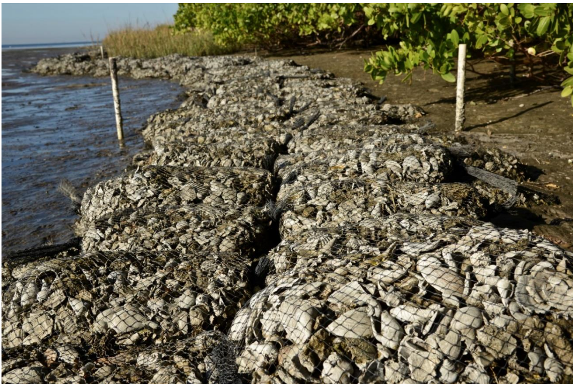
Figure 1.2 - Oyster Reefs formed using bags of shells along the shoreline at MacDill Air Force Base, Florida, USA (Pontee et al. 2016)
