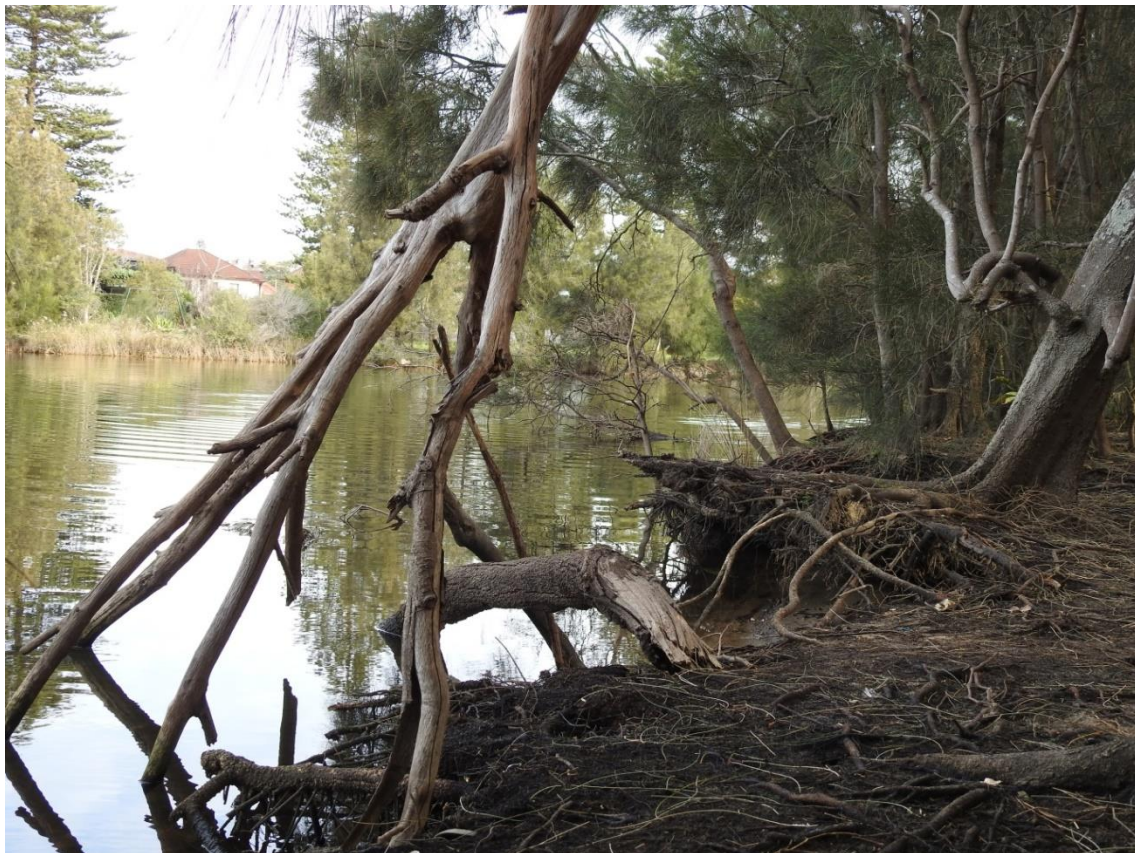
Figure 1.1 - Shoreline erosion of Manly Lagoon, NSW, Australia
