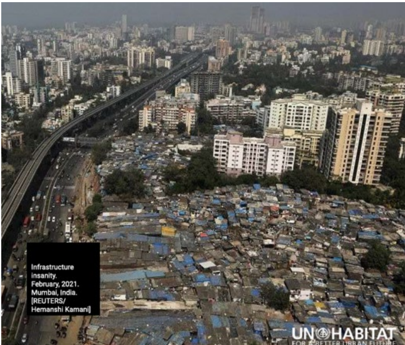
Figure 8 Infrastructure Insanity Mumbai India (UN Habitat, 2021)
