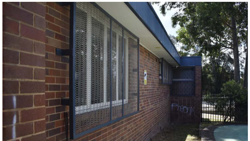
Figure 9. Security protections for ground-level windows.
