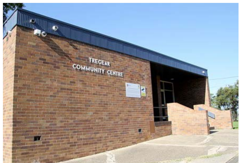
Figure 7. Northern view of Tregear community centre building.
