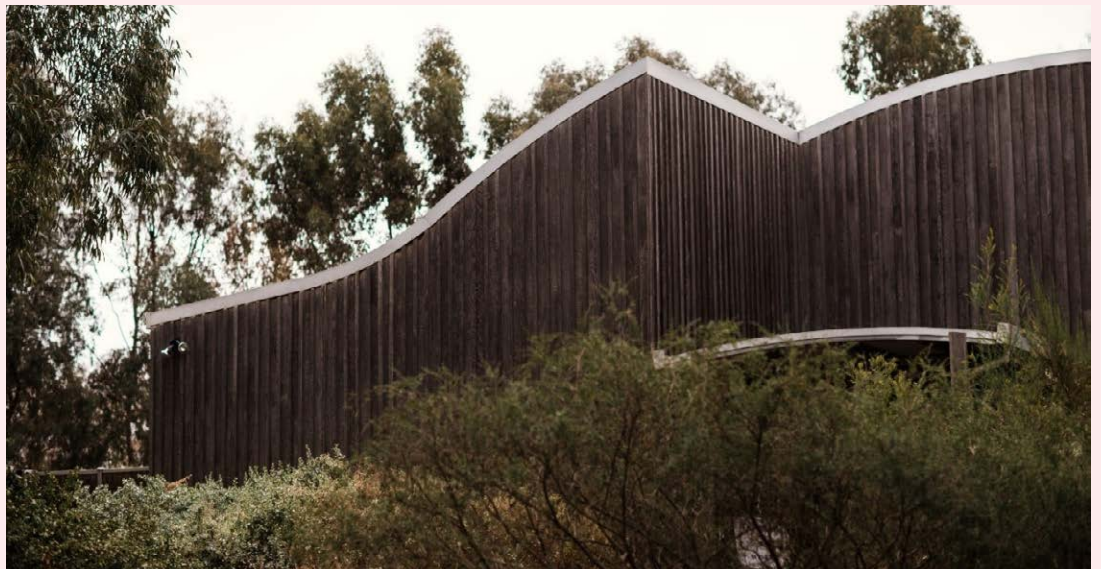
Fig. A3. Exterior views of the restaurant.
