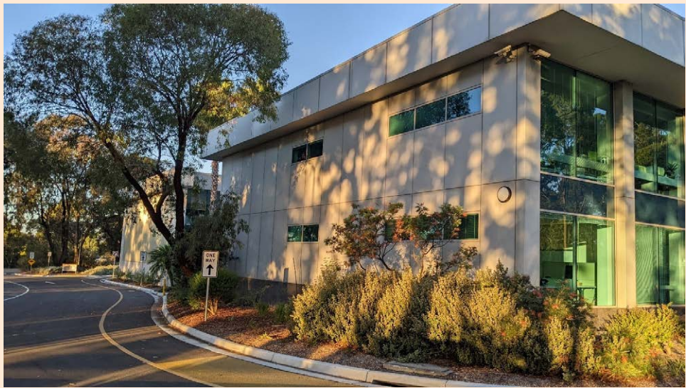
Fig. A5. Exterior view of the building.
