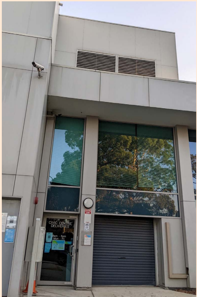
Fig. A4. Exterior view of the building.
