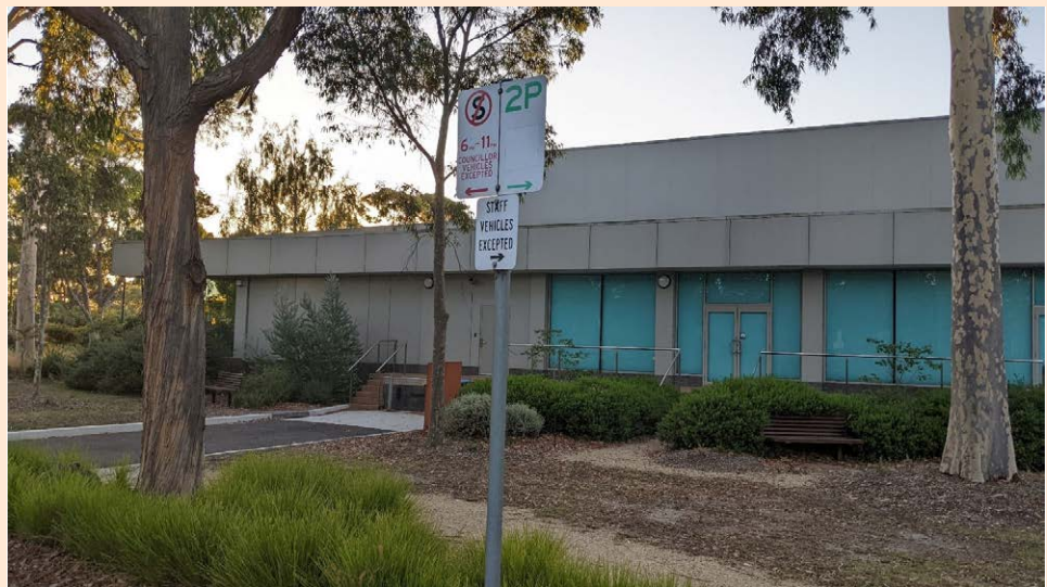
Fig. A8. Exterior view of the building.
