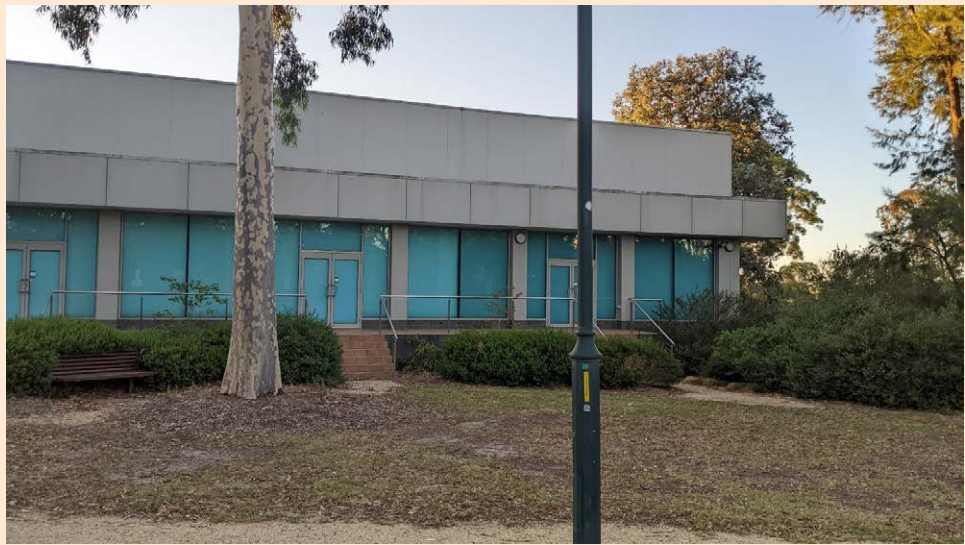
Fig. A7. Exterior view of the building.
