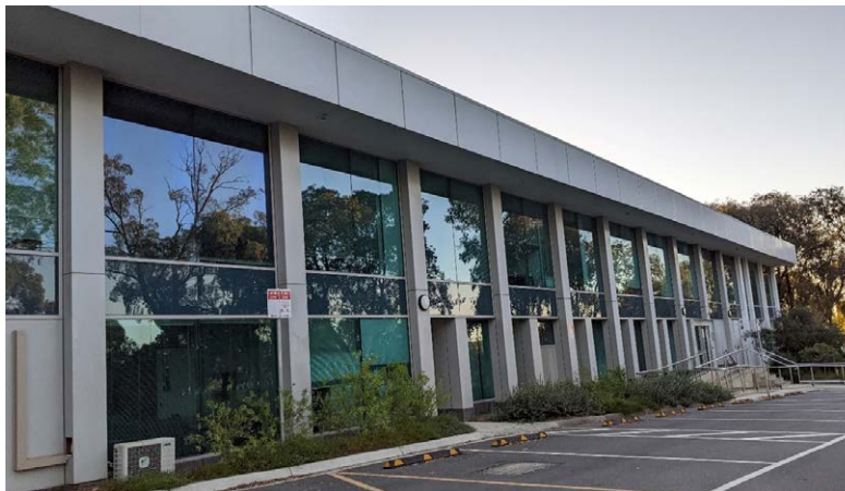
Figure 4. Northern view of Knox Civic Centre.
