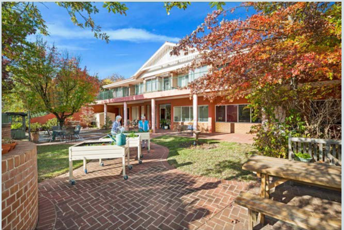
Fig. A3. Exterior view of the complex.
