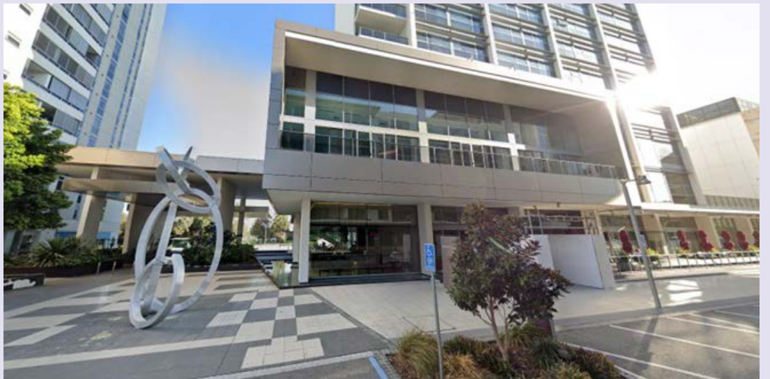
Fig. A3. Exterior view of the building.
