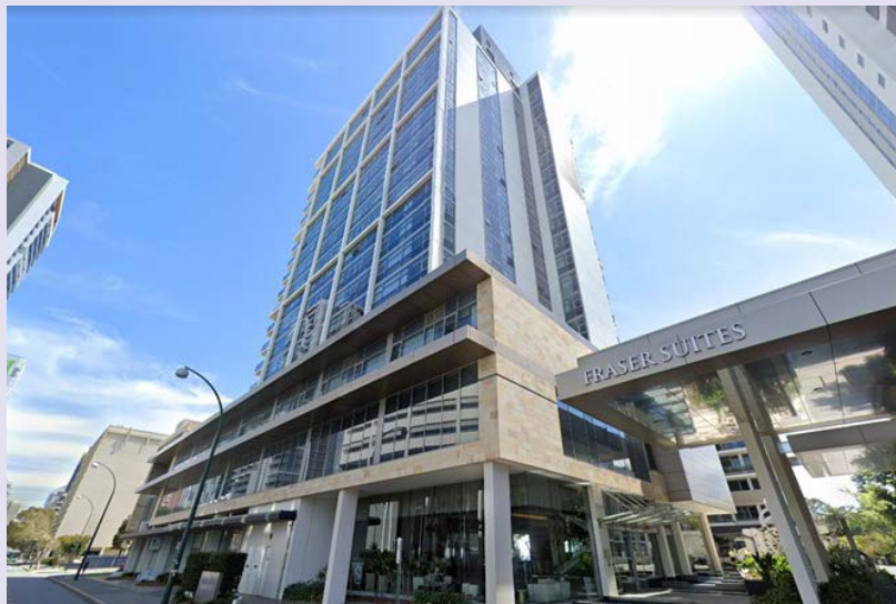
Fig. A1. Exterior view of the building.
