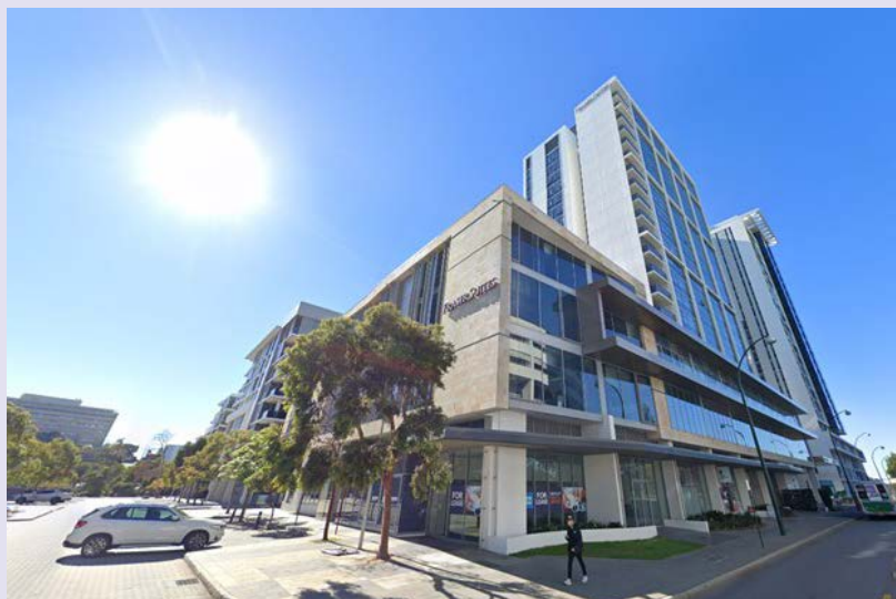
Fig. A2. Exterior view of the building.
