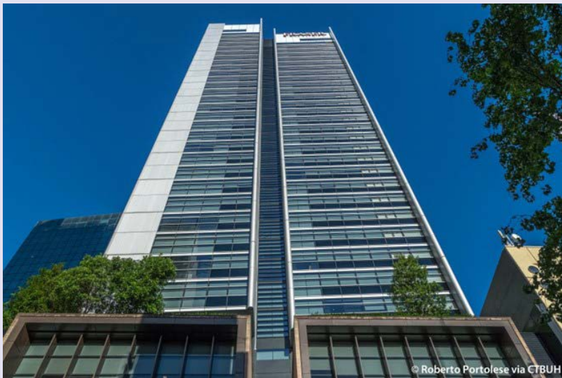
Fig. A3. Exterior view of the building.
