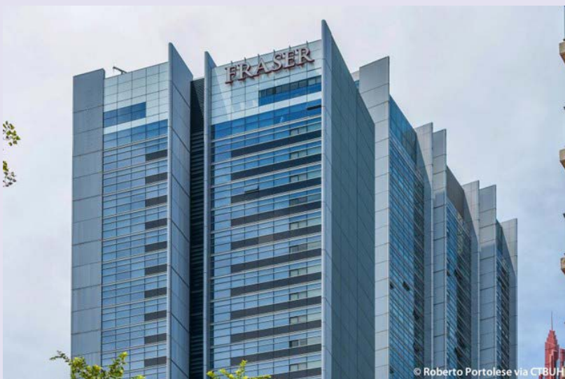
Fig. A4. Exterior view of the building.
