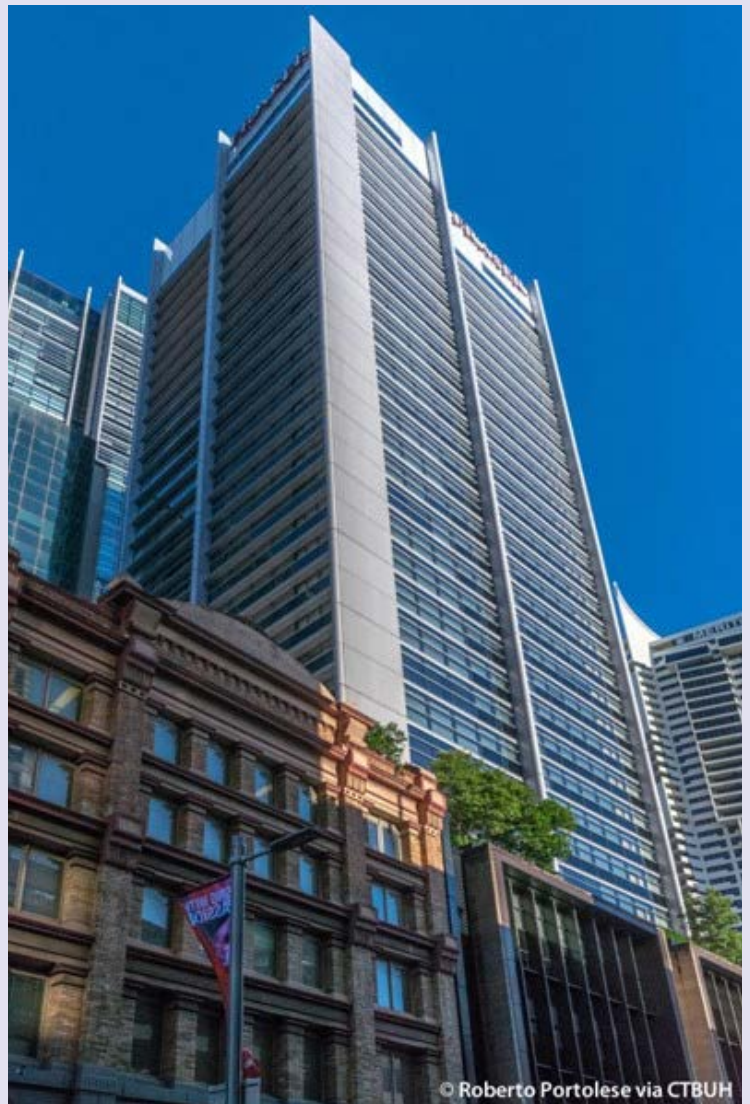
Fig. A2. Exterior view of the building.
