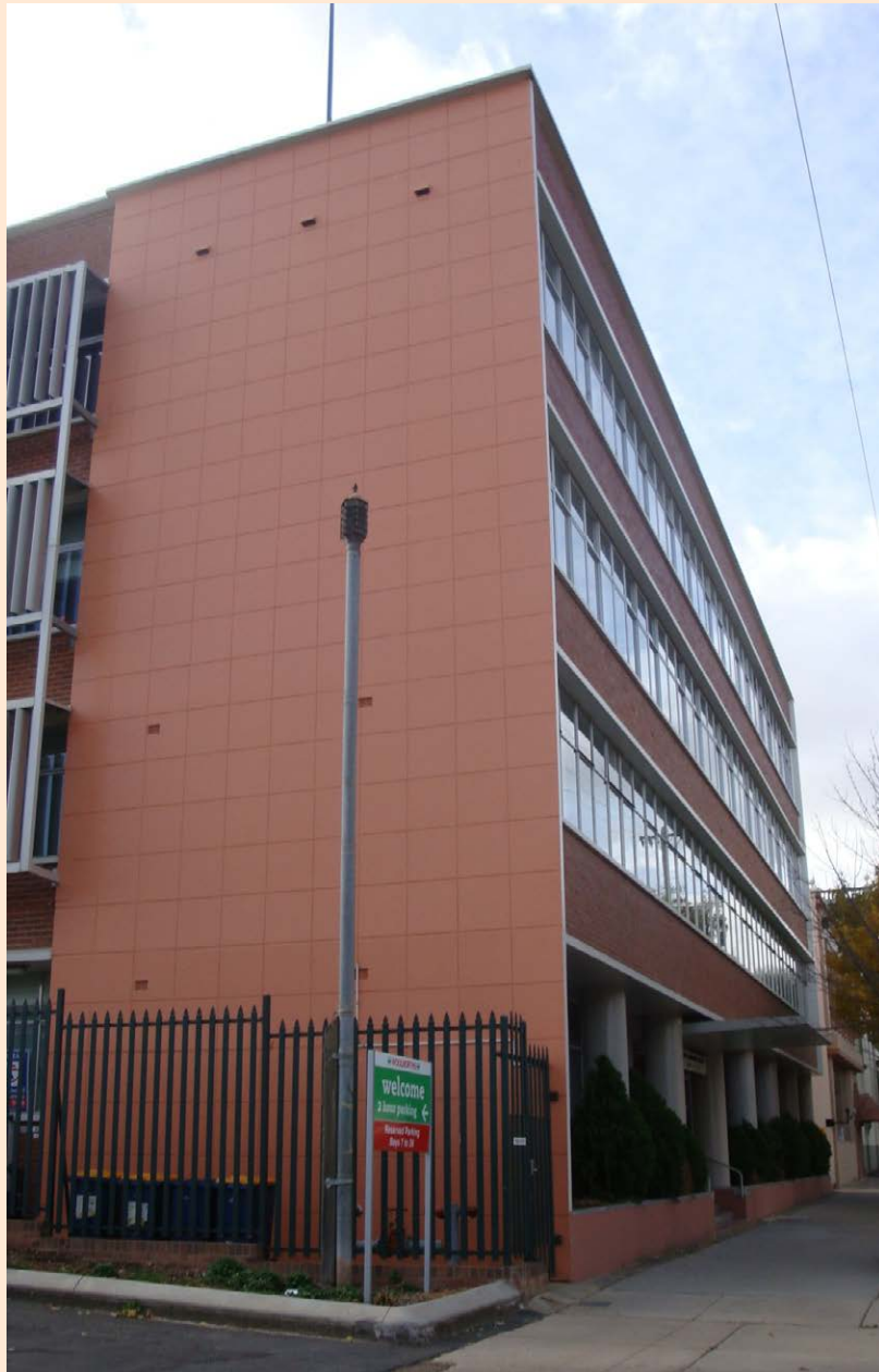
Fig. A2. Exterior Facade – South-West
