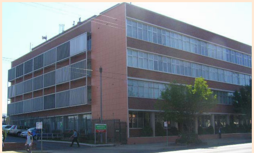
Figure 2. South-western view of 43-45 Johnston Street.
