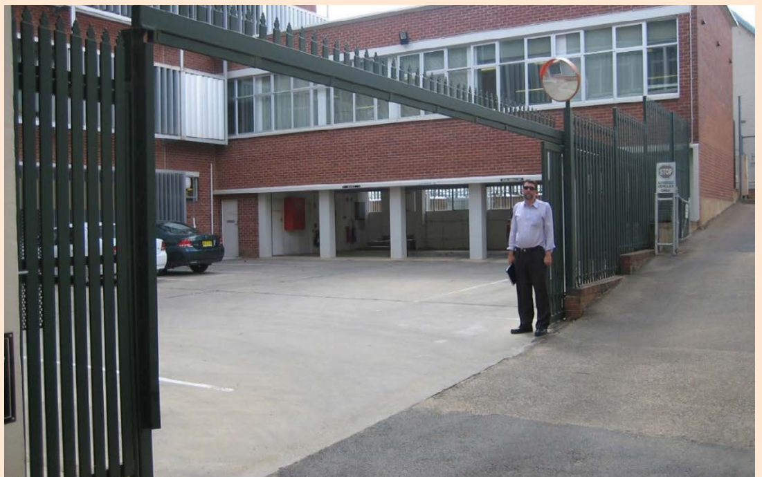
Fig. A6. Parking entrance
