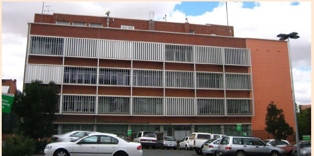
Fig. A3. Exterior Facade – West
