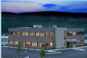
B03 New low-rise office building with roof insulation
