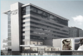
B16 Existing high-rise shopping mall centre
