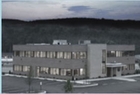
B13 Existing low-rise office building with roof insulation
