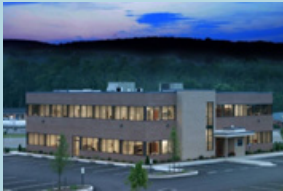
B01 Low-rise office building without roof insulation
