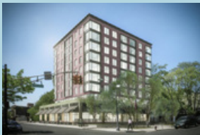
B04 New high-rise office building with roof insulation
