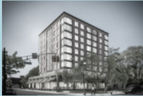
B14 Existing high-rise office building with roof insulation
