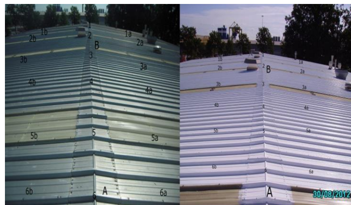
Figure 29 Cool Roof of the building, before/after
