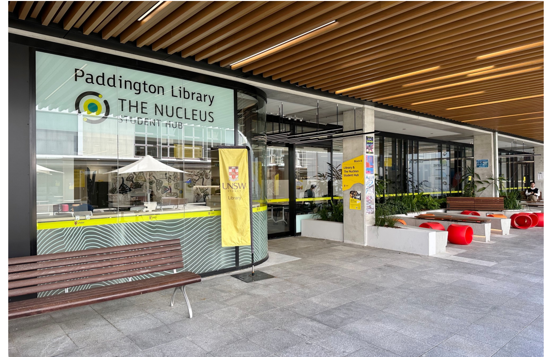
Entrance to Student Hub – Block D, Ground Floor
