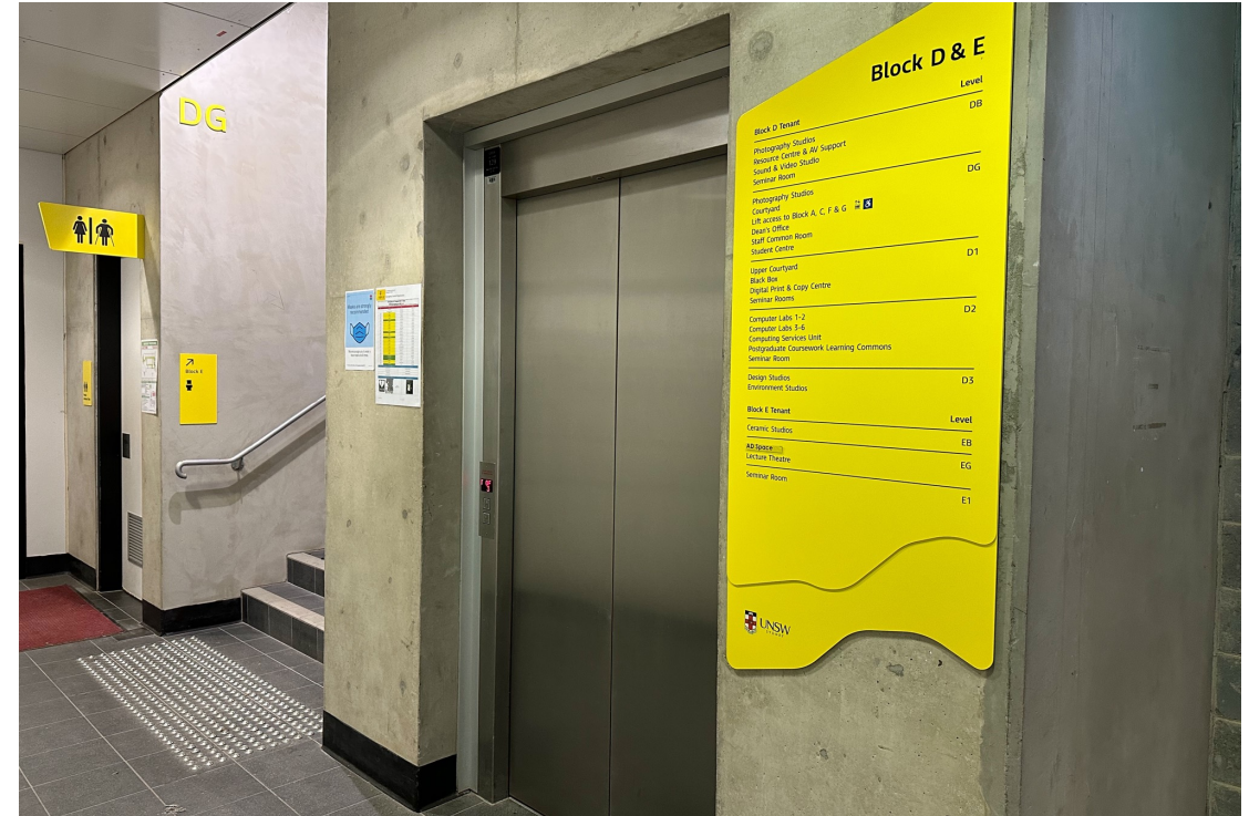
Elevator – Block D, Ground Floor
